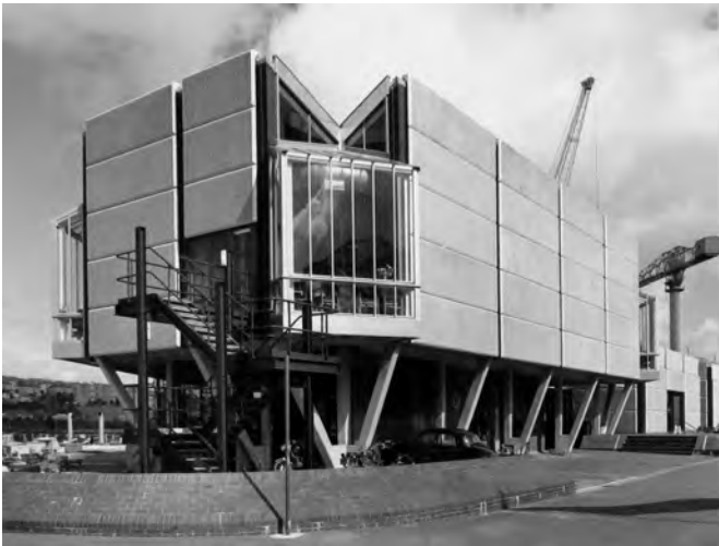
Fig. 129. NAAFI building (September 1979). TNA, CM 20/80 (1976). PSA: Devonport: Works Projects. Photograph albums. Fleet Maintenance Base Devonport: book no. 4. Reproduced with the permission of The National Archives.
