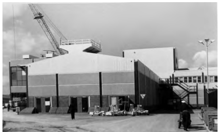
Fig. 128. Mast and Periscope Shop (September 1979). TNA, CM 20/80 (1976). PSA: Devonport: Works Projects. Photograph albums. Fleet Maintenance Base Devonport: book no. 4. Reproduced with the permission of the MoD.
