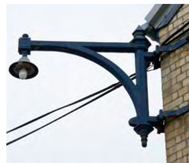
Fig. 184. DP13023. Devonport South Yard: photograph of Building S173 recorded before demolition. Cast iron lamp bracket on the southwest corner of S173 (8 Feb 2011). ©Historic England.
