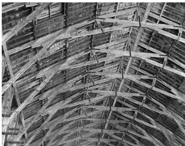
Above: Fig. 66. AA98/04662. Devonport Covered Slip No. 1 (1774–75) photograph by Eric de Mare showing the roof timbers added in the nineteenth century (1956). The only remaining intact eighteenth century slip within a royal dockyard (Coad, 1989, p. 197). Reproduced by permission of Historic England.
