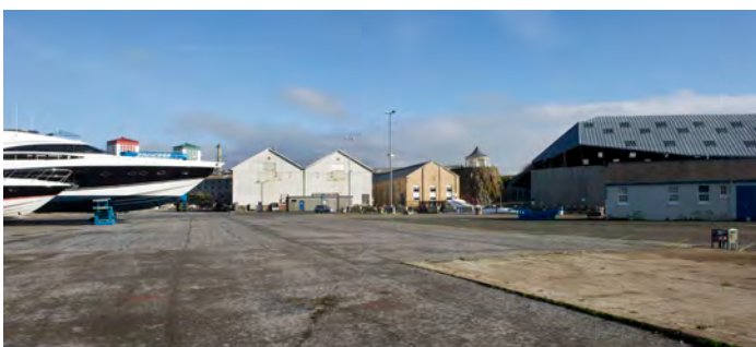
Fig. 181. DP130113. Devonport South Yard: photograph of Building S173 recorded before demolition. General view looking northeast across the dockyard towards S172 and S173 (8 Feb 2011). King's Hill Gazebo (1822, S186) and the newly roofed Covered Slip No. 1 are on the right. S173 was constructed as a Plumbers' Shop as part of the project dating from 1900 to supply the building of Dreadnoughts on nearby Slip No. 3 (English Heritage, Aug 2010, Listing Advice Report Building S173). Princess Yachts vessels are seen on the left. ©Historic England.
