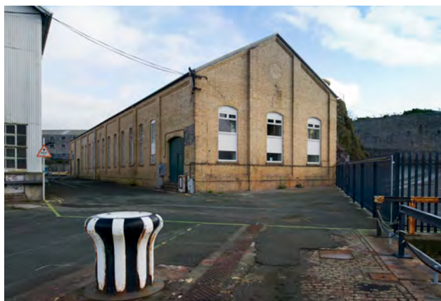
Fig. 182. DP130116. Devonport South Yard: photograph of Building S173 recorded before demolition. View of S173 looking towards the west end doorway on the west elevation (8 Feb 2011). King's Hill Gazebo (1822, S186) can just be seen behind it to the right, with new fencing to secure Princess Yachts' land. Shallow Dock is in the bottom right hand corner. ©Historic England.
