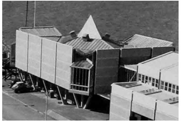
Fig. 130. NAAFI building, September 1979. Detail from Fig. 125. TNA, CM 20/80 (1976). PSA: Devonport: Works Projects. Photograph albums. Fleet Maintenance Base Devonport: book no. 4. Reproduced with the permission of The National Archives.
