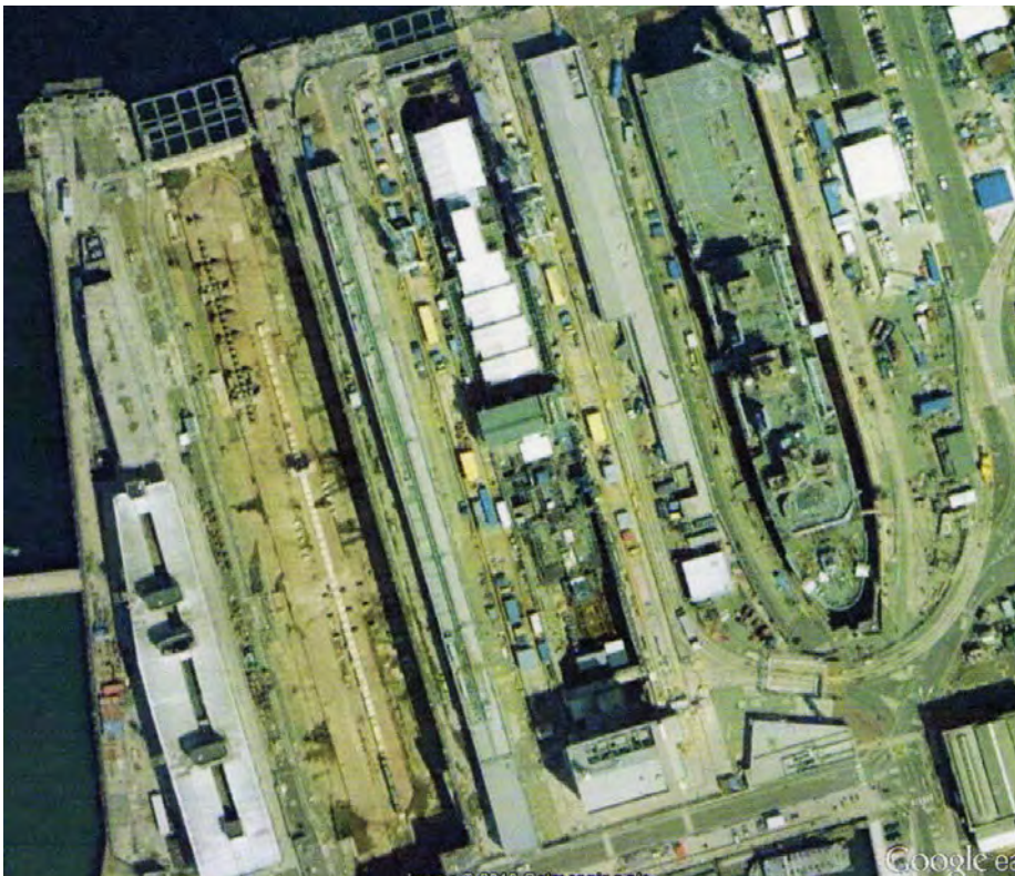
Fig. 180. Google aerial photograph of Devonport Dockyard. Retrieved from Google Earth in 2013.
