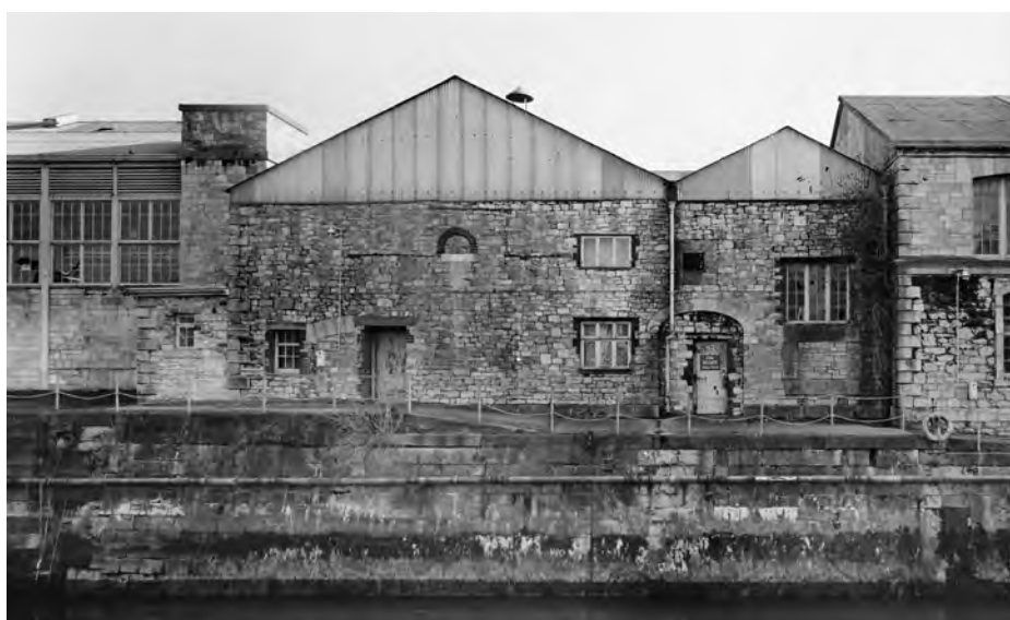
Fig. 70. BB96/03891. Devonport South Yard South Smithery (S126) photograph of north elevation of centre building (29 Feb 1996). ©Crown copyright.HE.
