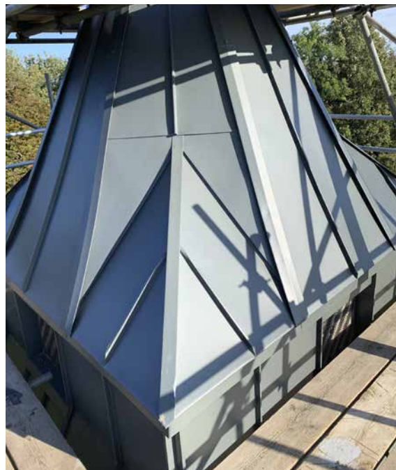
Photo: Zinc covering on a church spire © Bakers of Danbury
