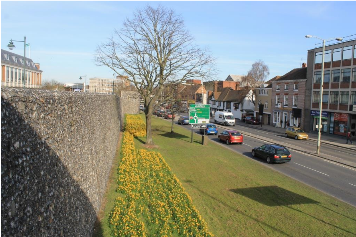
Fig. 2 Canterbury City Walls at Upper Bridge Street (SE of the city) from one of 13 original bastions
