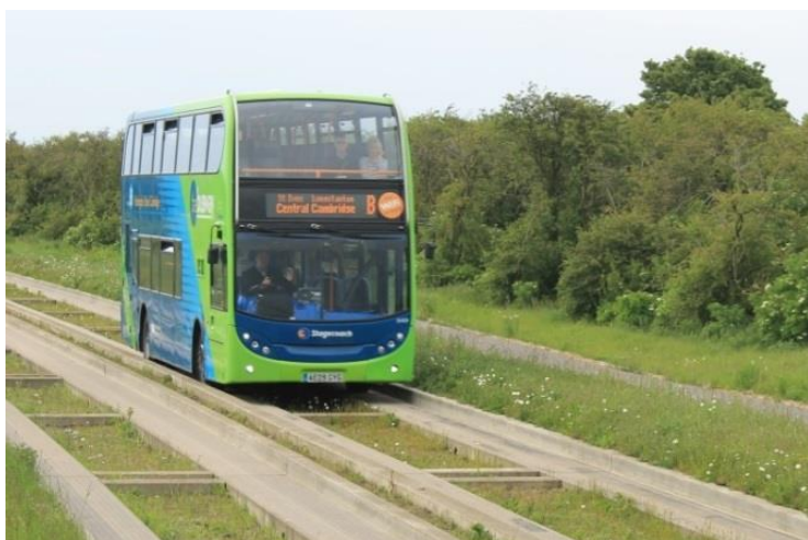
Guided Busway in use near Longstanton
