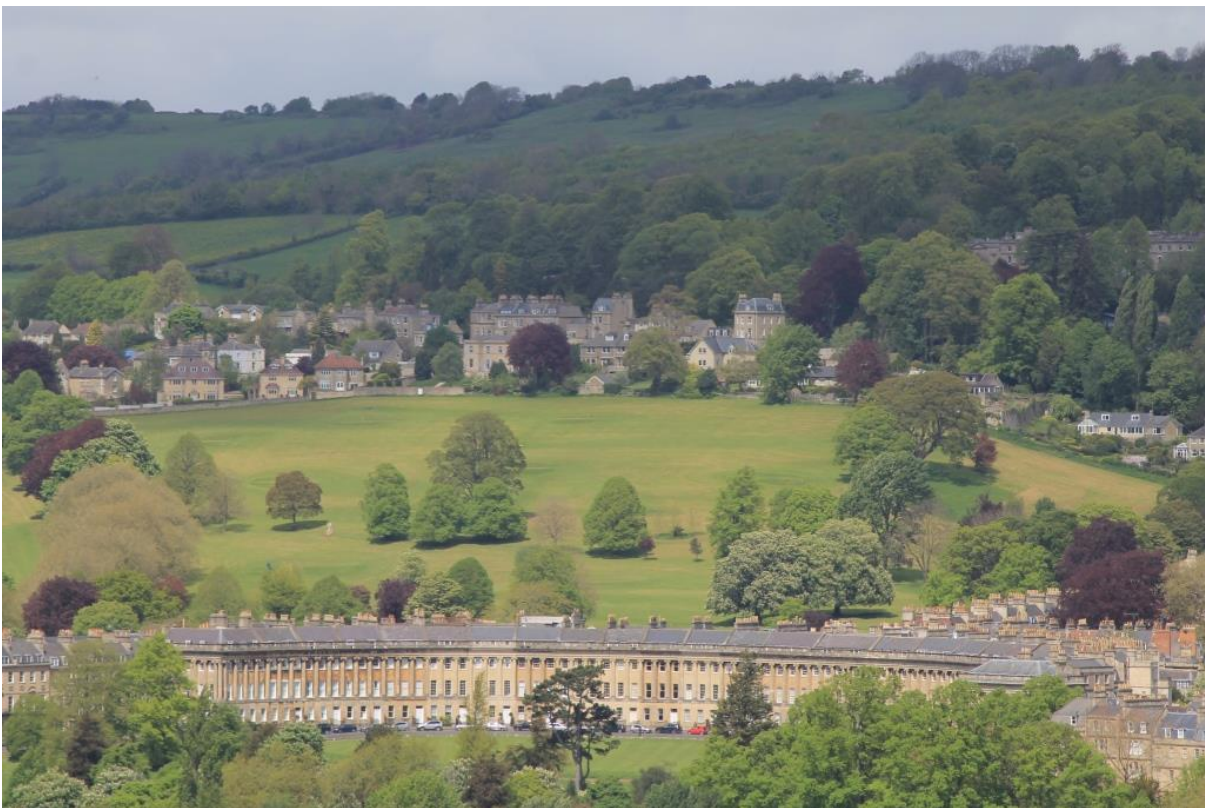
The Royal Crescent, seen from Beechen Cliff, highlights its green space context, with open space in front, an approach golf course behind, and undeveloped countryside on the steeper slopes of Primrose Hill above
