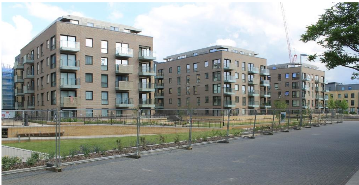
Apartment blocks in the CB1 development near the railway station, with the gardens too almost complete.
