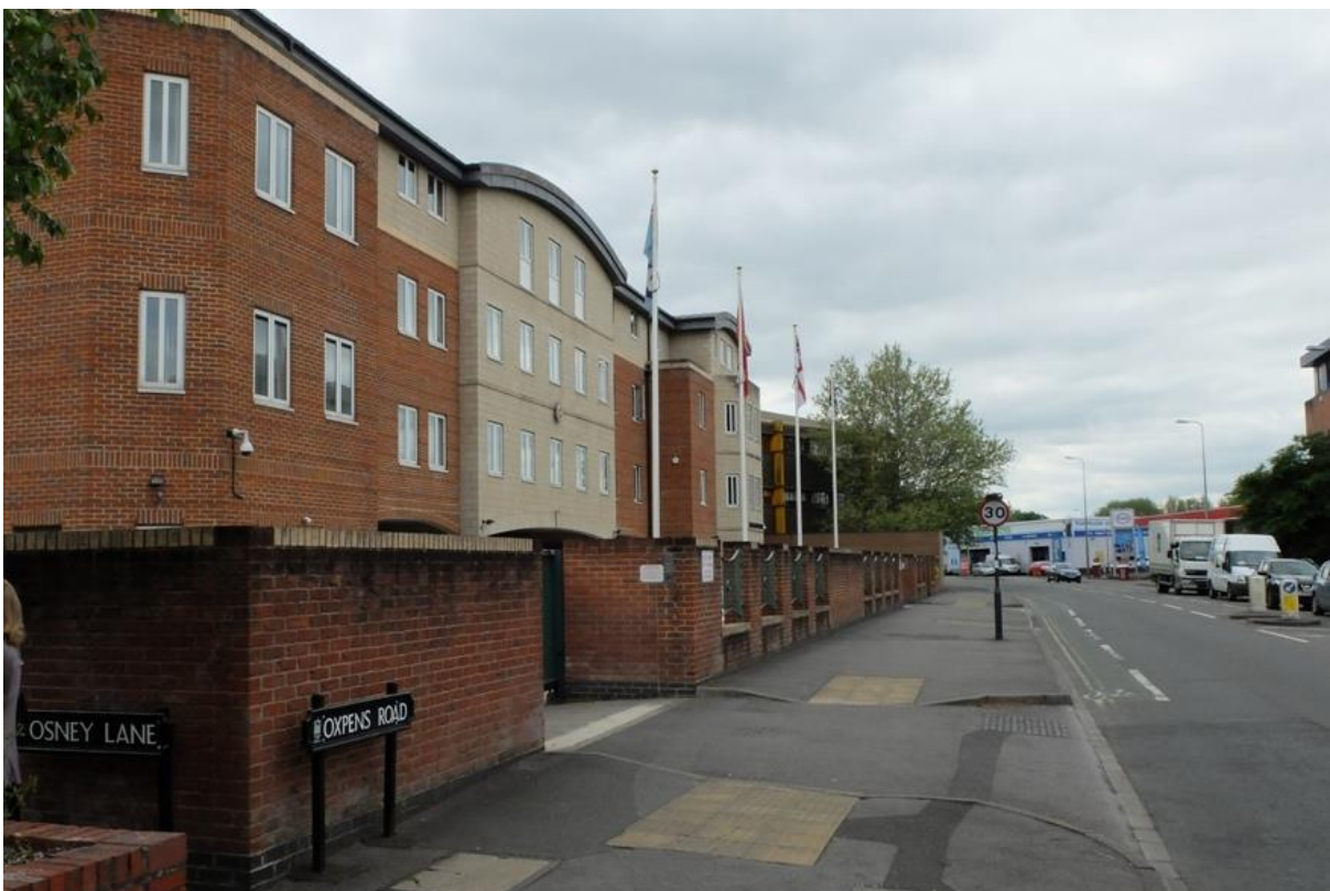
Not far from the city centre, The Oxford University Royal Naval Unit seems to show how far the public sector commissioning process has moved away from a culture which produced the exquisite architecture of the Royal Naval College at Dartmouth
