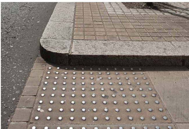
Integrated tactile paving at a lowered crossing.
