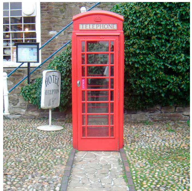
A K6 kiosk given pride of place in an open space. Note the smooth natural stone setts inserted into an area of cobbles to facilitate access.
