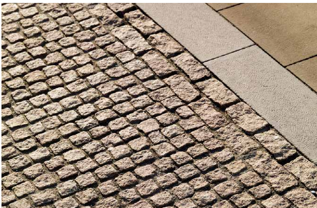
Reinstated traditional paving in Sheffield.
