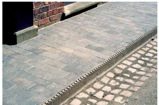
Historic paving accurately recreated.
