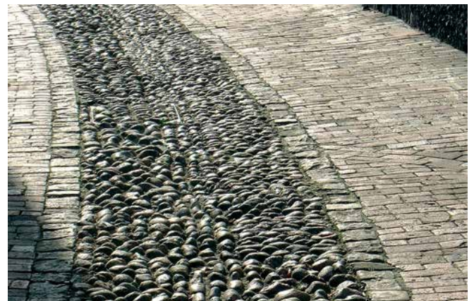
A combination of local river cobbles and brick paviours.
