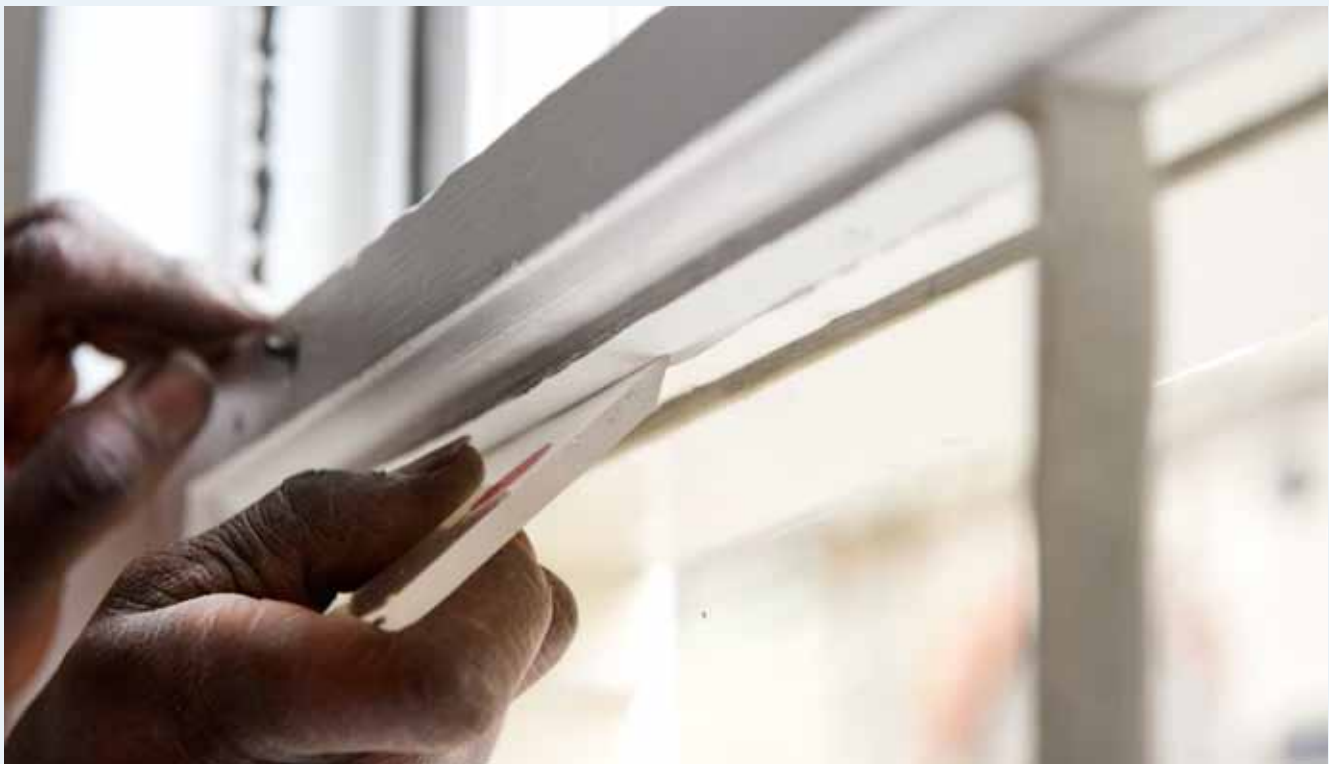
Installing secondary glazing panels to the English Heritage office in Swindon, Wiltshire. Photo by James O. Davies, © English Heritage.
