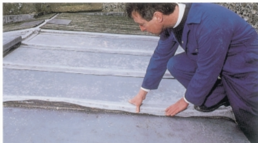
Figure 27 Replacing the lead
