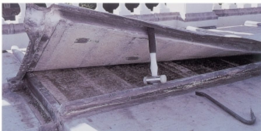
Figure 26 A sheet with its corner raised and propped
