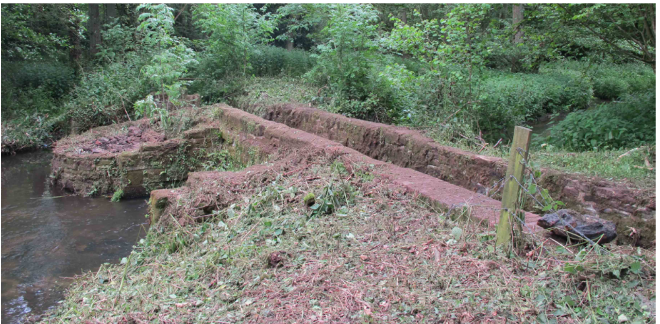
Figure 13 Aqueducts carried water through narrow sections of the Wey Valley, allowing its water meadow systems to function in difficult topography. This example at Bramshott Court is one of several built to connect water meadows on either side of the river.
