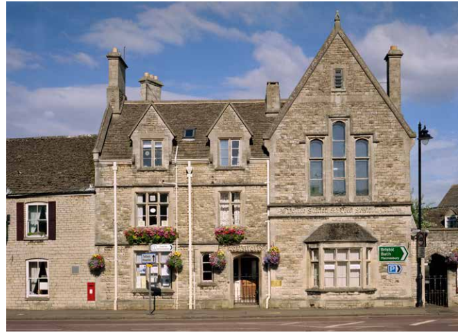
Figure 23 The exterior of the former Police Station and Petty Sessions Court at Tetbury, Gloucestershire, 1884, by James Medland. This is one of a group of combined police stations and magistrates' courts, constructed in Gloucestershire in stone in a Gothic style to match local buildings. Listed Grade II.
