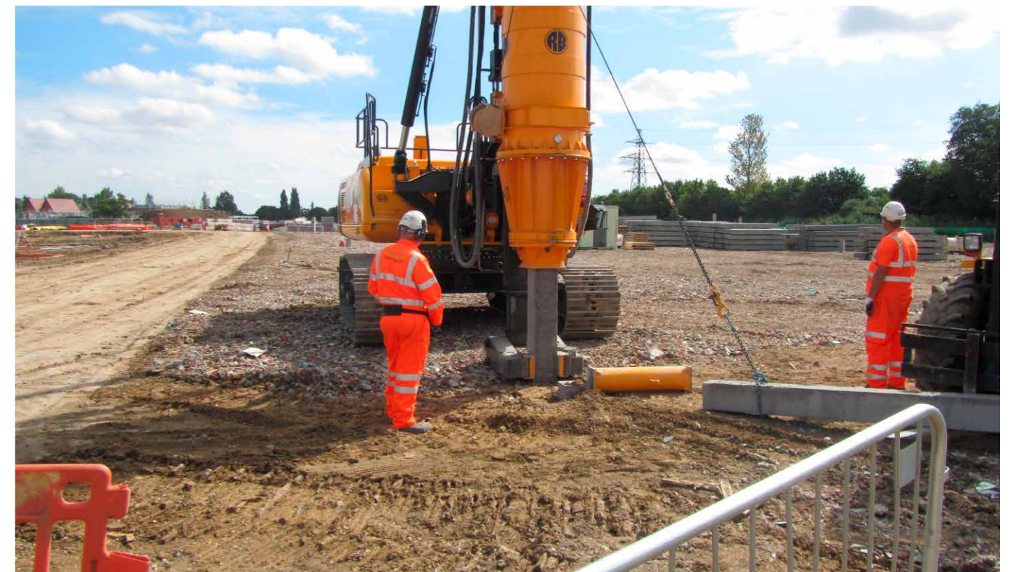
Above: Installing sections of a preformed concrete pile. © Roger Bullivant Limited
