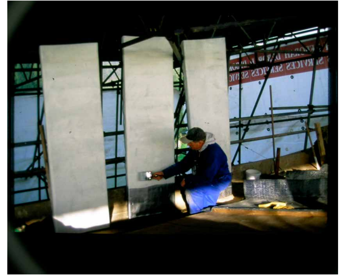
A simple mixture of chalk powder and water ('chalk slurry') painted onto the underside proved to be effective
