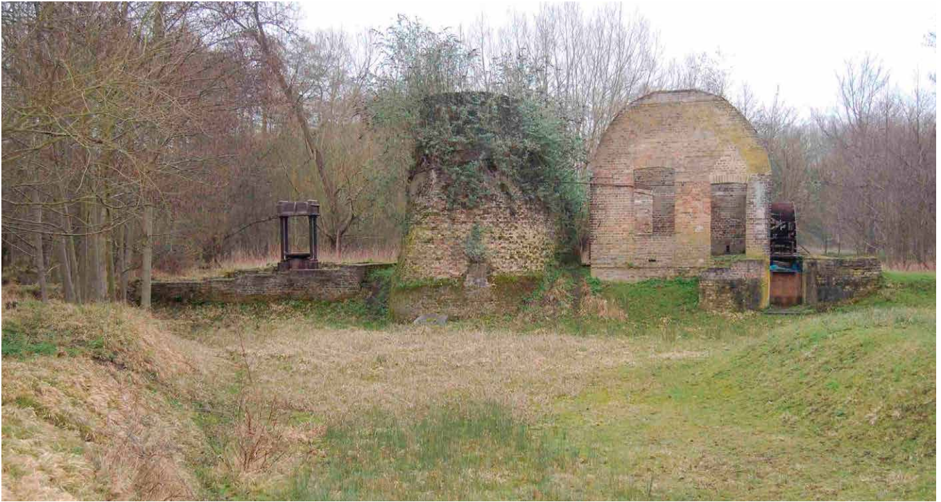
Figure 13 Royal Gunpowder Factory, Waltham Abbey, Essex. A unique mid-nineteenth century gunpowder hydraulic press house with a surviving waterwheel, pump and press, probably manufactured by William Fairbairn
