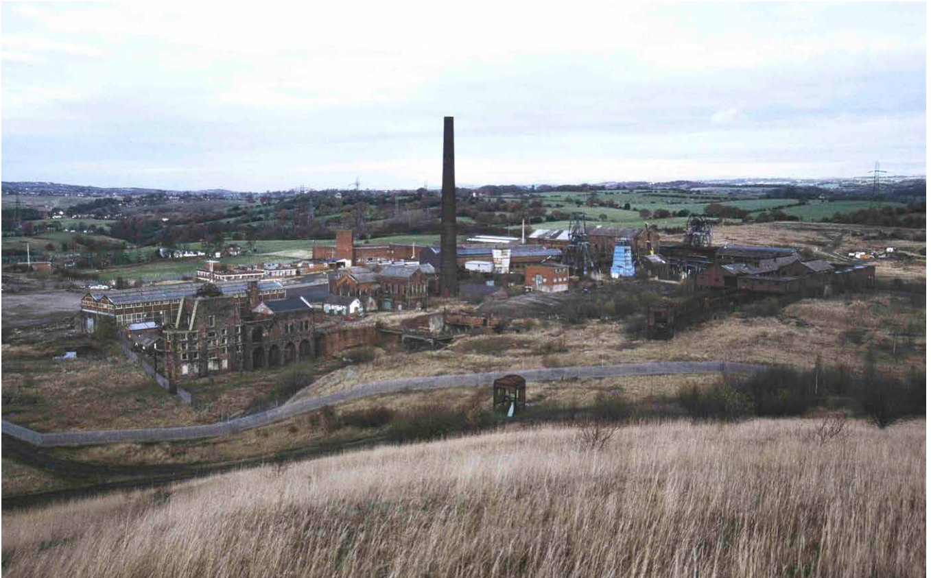
Figure 9 Chatterley Whitfield colliery, Stoke-on-Trent, Staffordshire, was one of England's most productive in the later nineteenth and earlier twentieth century, finally closing in 1977. A period as a museum meant,
