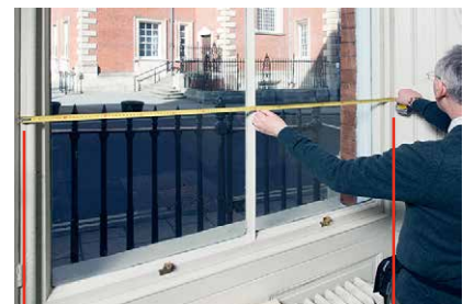
Measuring between splays
