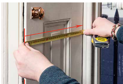
A Measuring the splay
