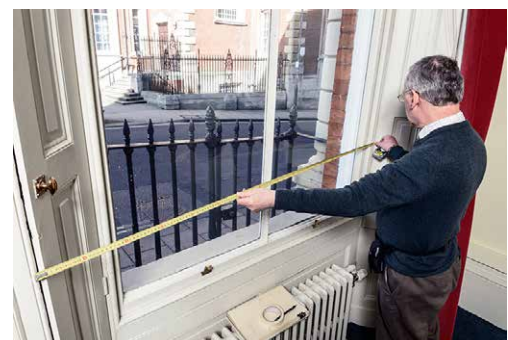
Measuring the diagonal of the opening
