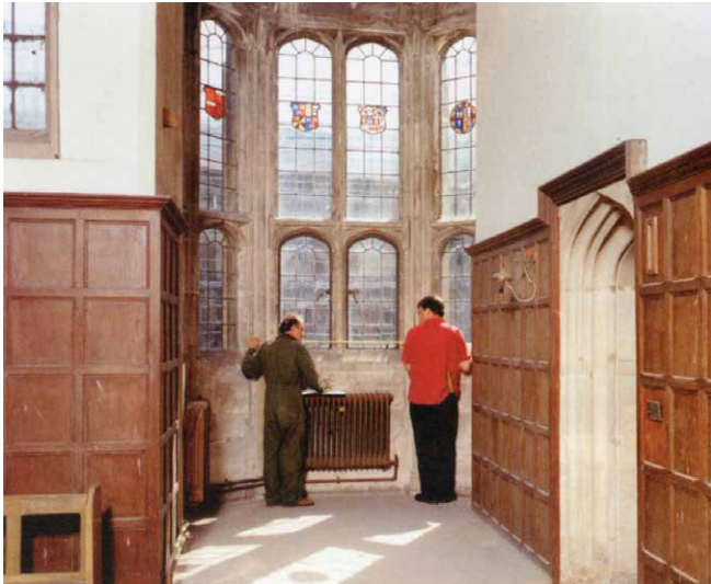
Figure 2 Measuring by hand involves intimate contact with the building and can greatly enhance the information gleaned from a site. It is particularly effective when combined with TST surveying.
