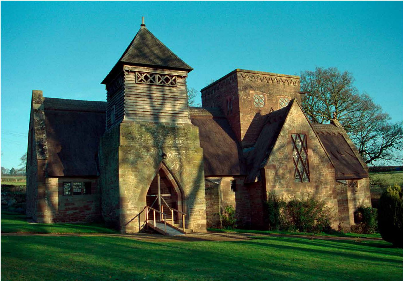
Figure 9 Something of a technological wolf in sheep's clothing, the traditional thatch of All Saints', Brockhampton, Herefordshire, disguises a concrete roof. Designed by
