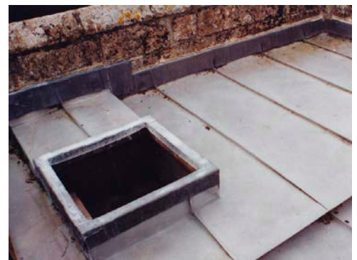
Figure 4: Lead used for flashings and access hatch capping
