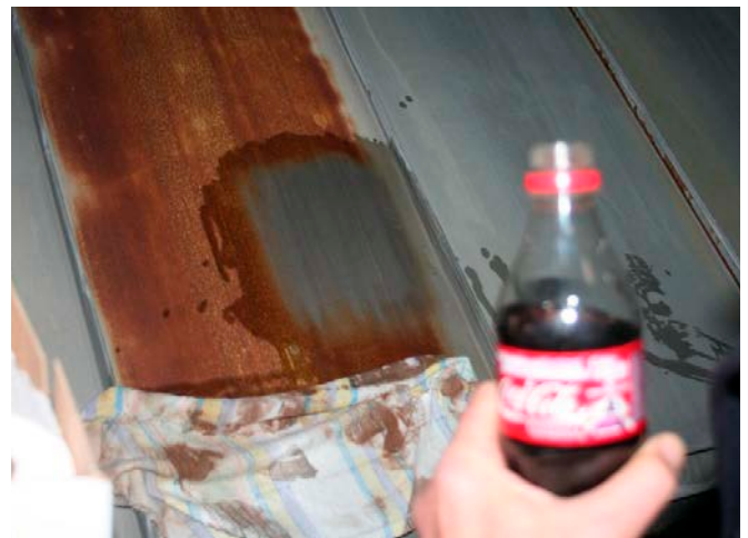
Figure 13: Stain successfully removed using weak phosphoric acid solution
