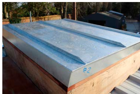
Figure 5: Standing-seam roof sample under test
