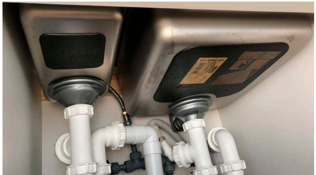
Figure 7: Mats bonded to underside of sink to reduce dripping noises
