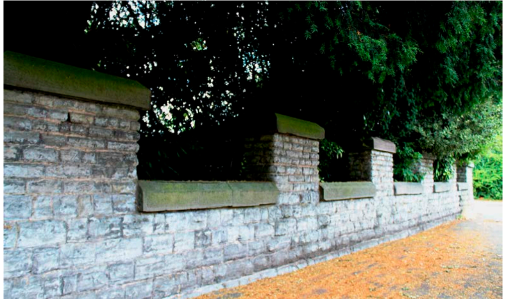
Figure 24: Boundary wall, Worcester Crematorium. Blue Lias.
