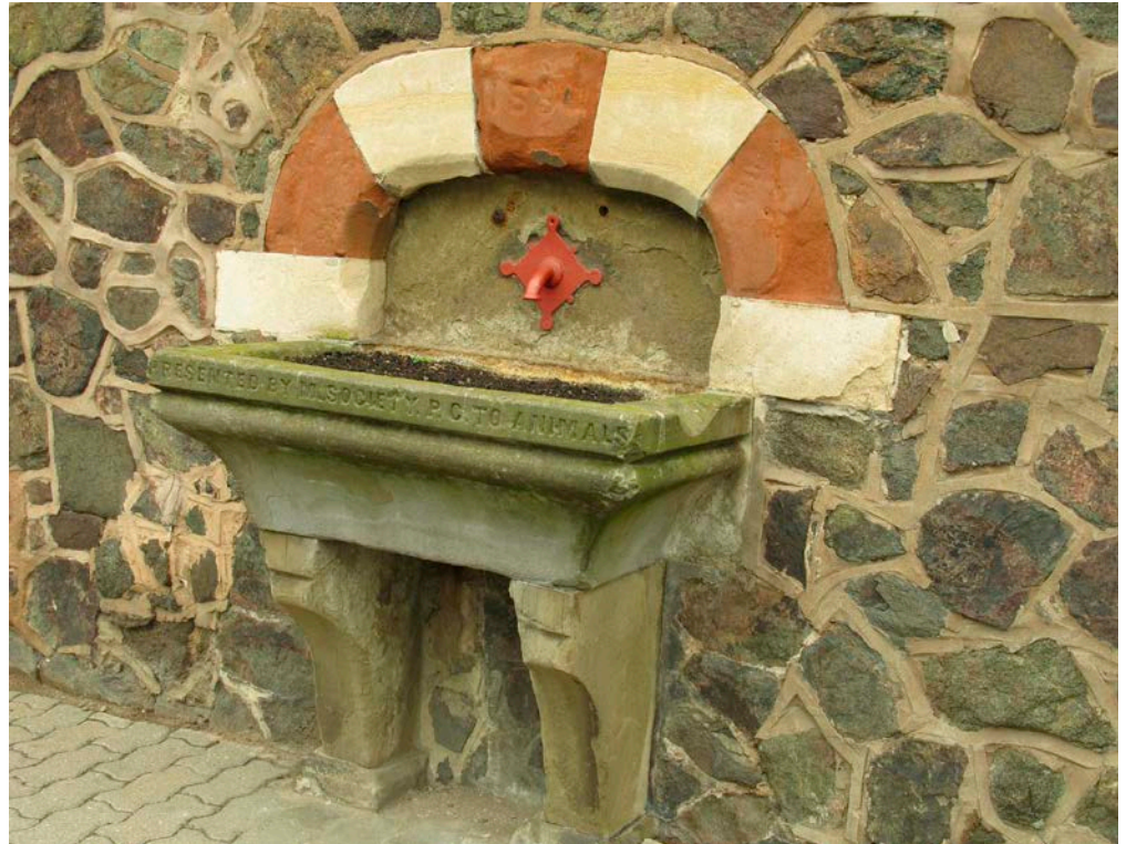
Figure 3: Drinking trough, Great Malvern station. Highley Sandstone with arch of Cotswold Stone and red Bromsgrove Sandstone in a wall of Malvern Stone.
