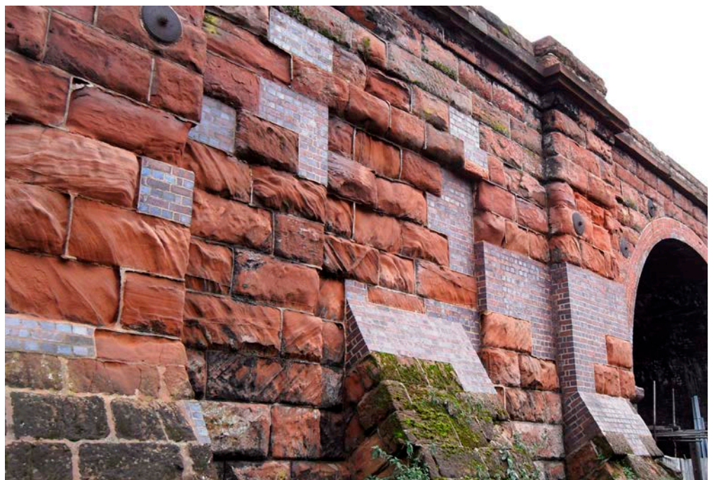
Figure 18: Railway viaduct, Bewdley. Bridgnorth Sandstone.
