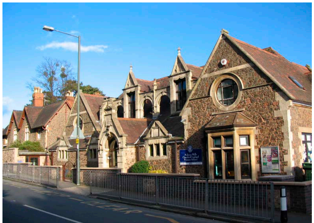
Figure 4: Malvern Wells Church of England Primary School. Malvern Stone rubble walls and Cotswold Stone dressings.
