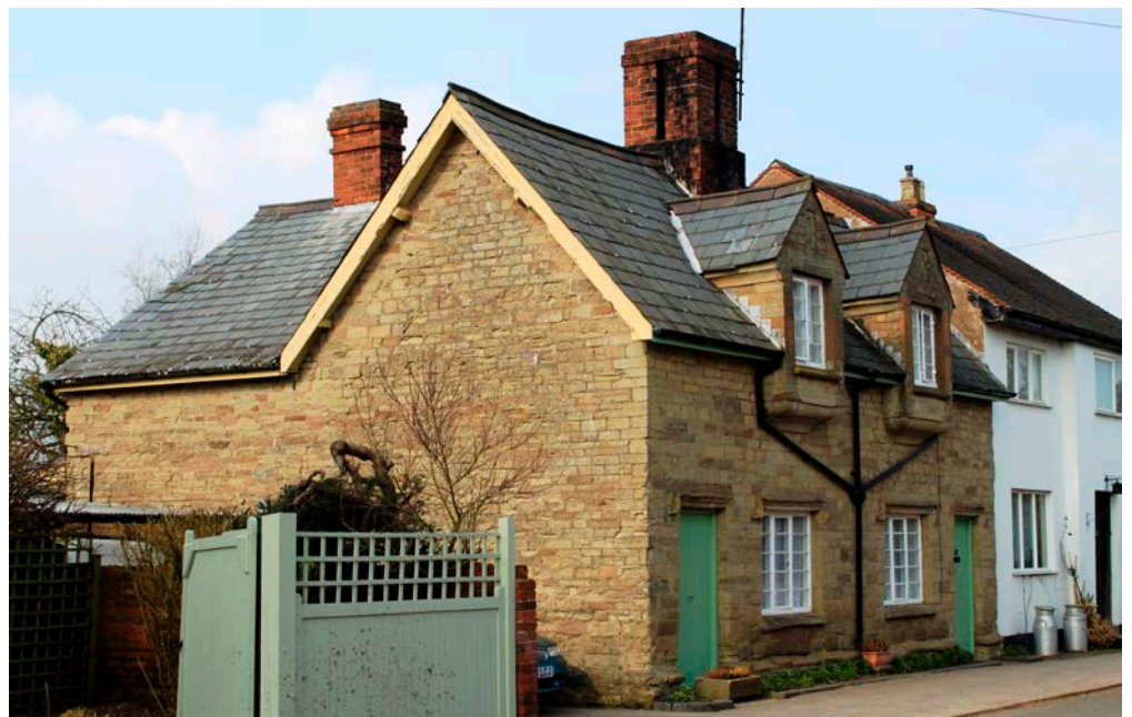
Figure 6: Cottage, Clifton upon Teme. St Maughans Formation sandstone rubble.
