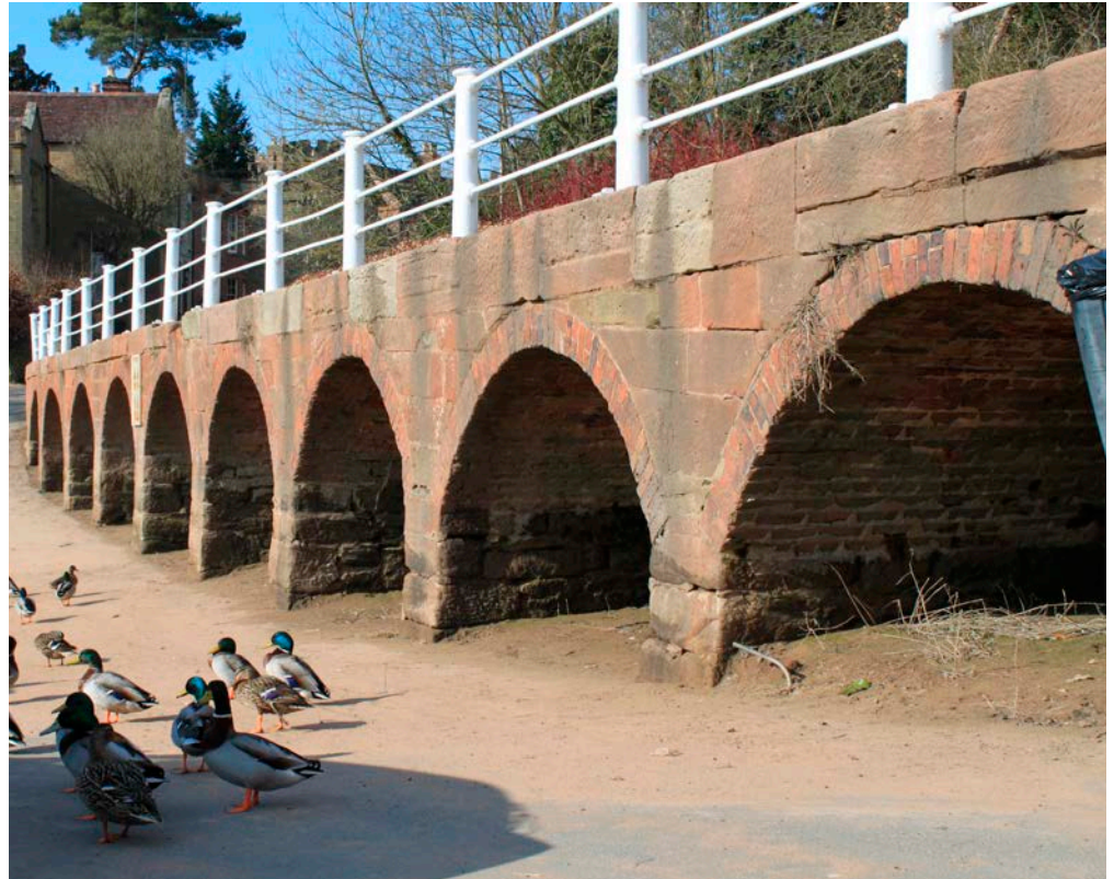
Figure 16: Arley quayside. Alveley Stone.
