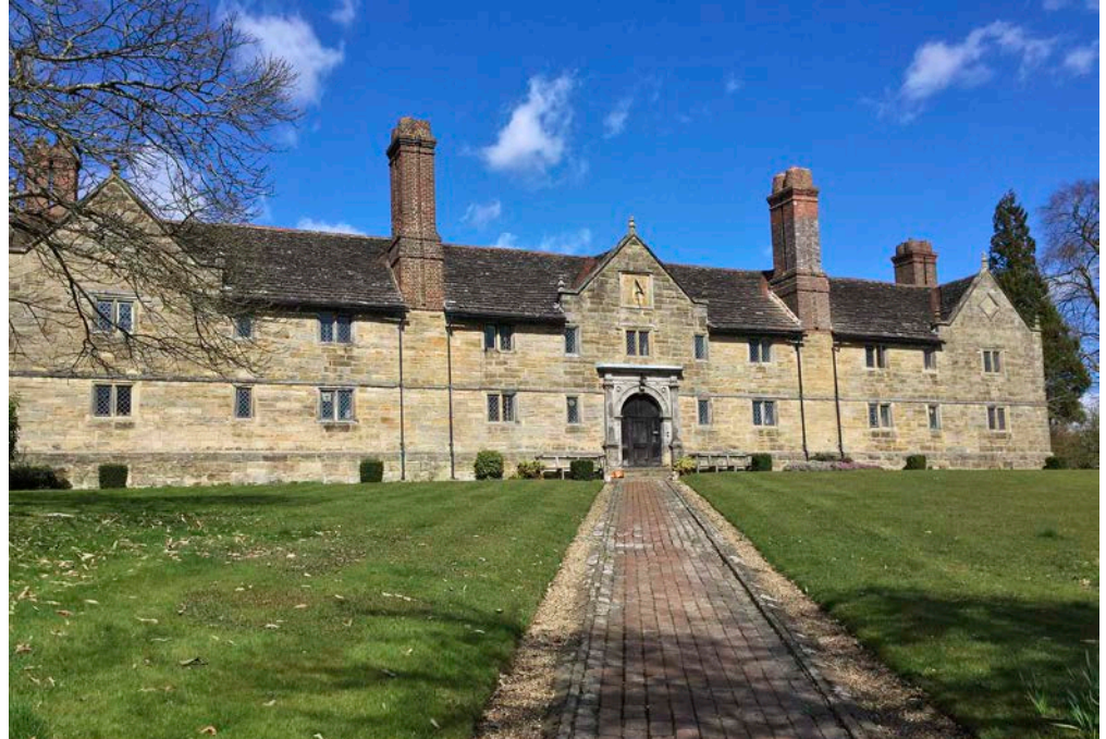
Figure 3: Almshouses, Sackville College, East Grinstead. Lower Tunbridge Wells Sandstone, Ardingly Sandstone, and Horsham Stone slate roof.
