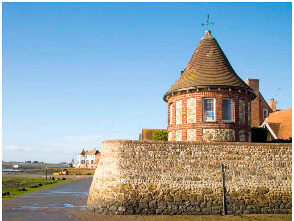
Figure 25: Quayside walls, Bosham Harbour. London Clay Cementstone.
