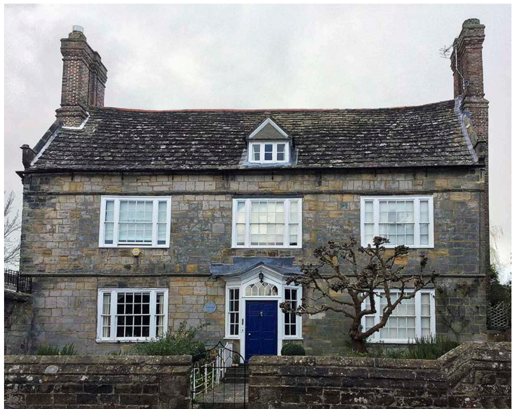
Figure 5: Manor House, High Street, Cuckfield. Ardingly Sandstone and Horsham Stone slate.
