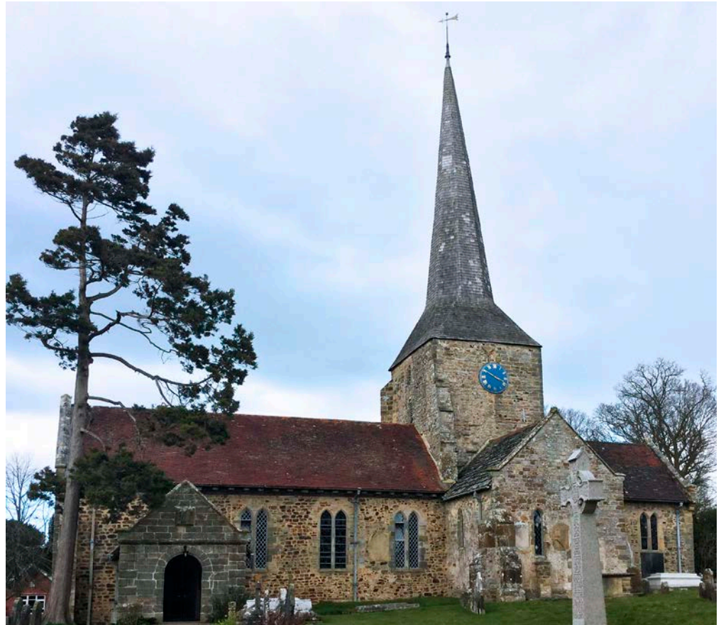
Figure 2: St Giles Church, Horsted Keynes. Ashdown Sandstone and Ardingly Sandstone, and part Horsham Stone slate roof.
