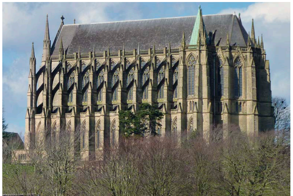
Figure 6: Lancing College Chapel, Lancing. Cuckfield Stone with Ardingly Sandstone and Bath Stone.
