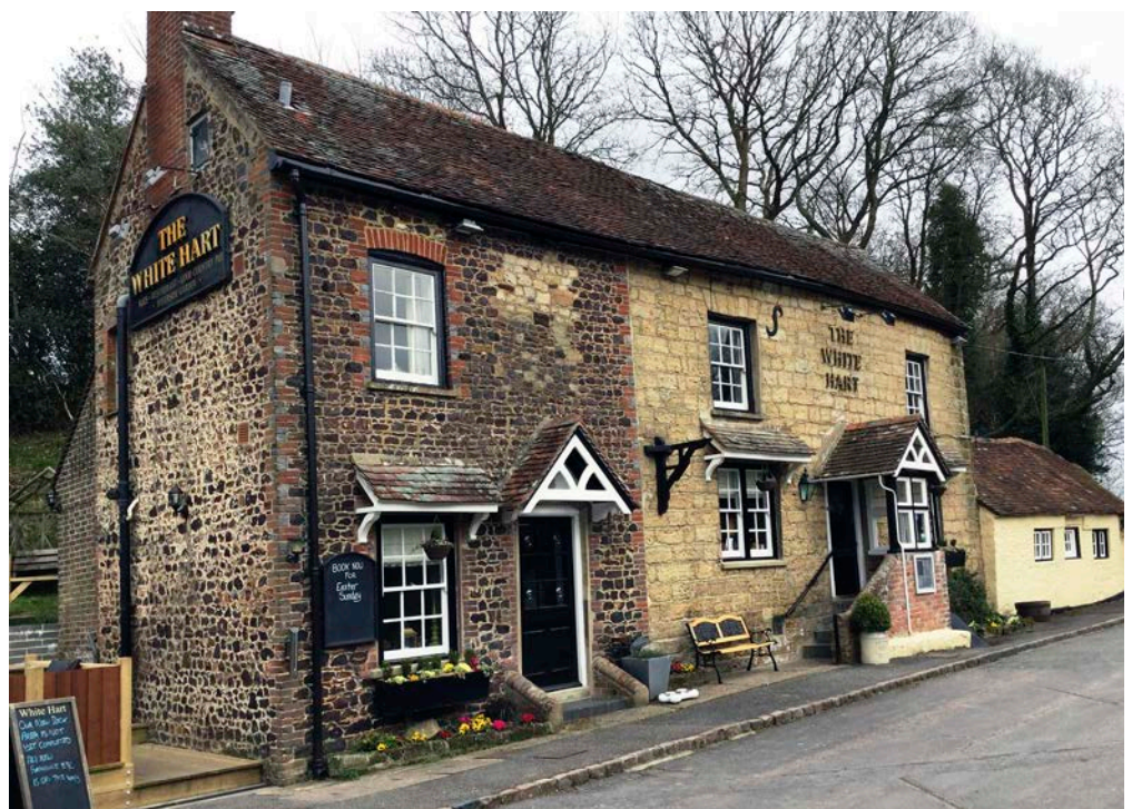
Figure 15: Public house, Pulborough. Carstone and Hythe Sandstone.
