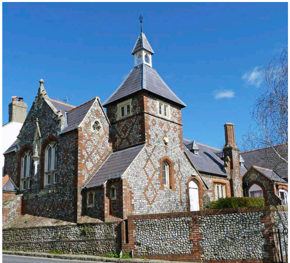
Figure 19: Old School House, Angmering. Flint.
