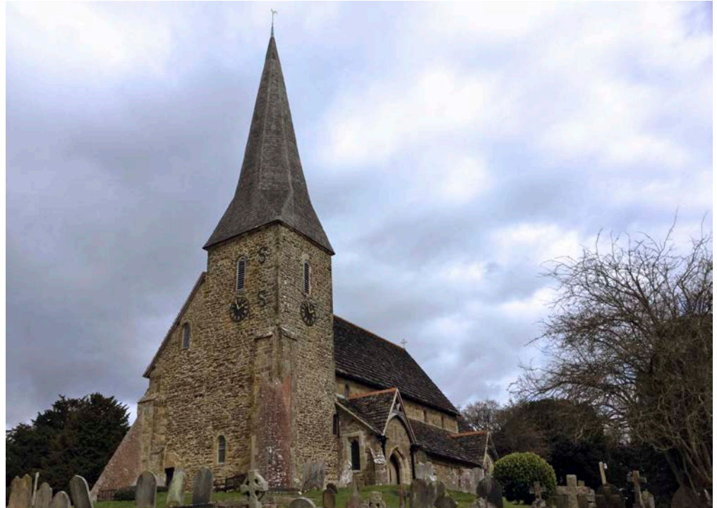
Figure 10: St Peter's Church, Wisborough Green. Billingshurst Sandstone with Horsham Stone slate roof.
