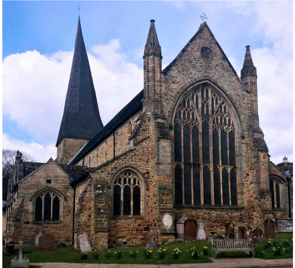
Figure 9: St Mary's Church, Horsham. Horsham Stone and Ardingly Sandstone, with Horsham Stone slate roof.
