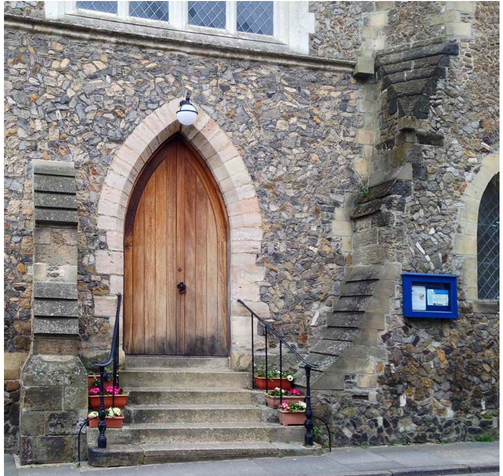
Figure 13: United Reform Church, Petworth. Hythe Chert random rubble.
