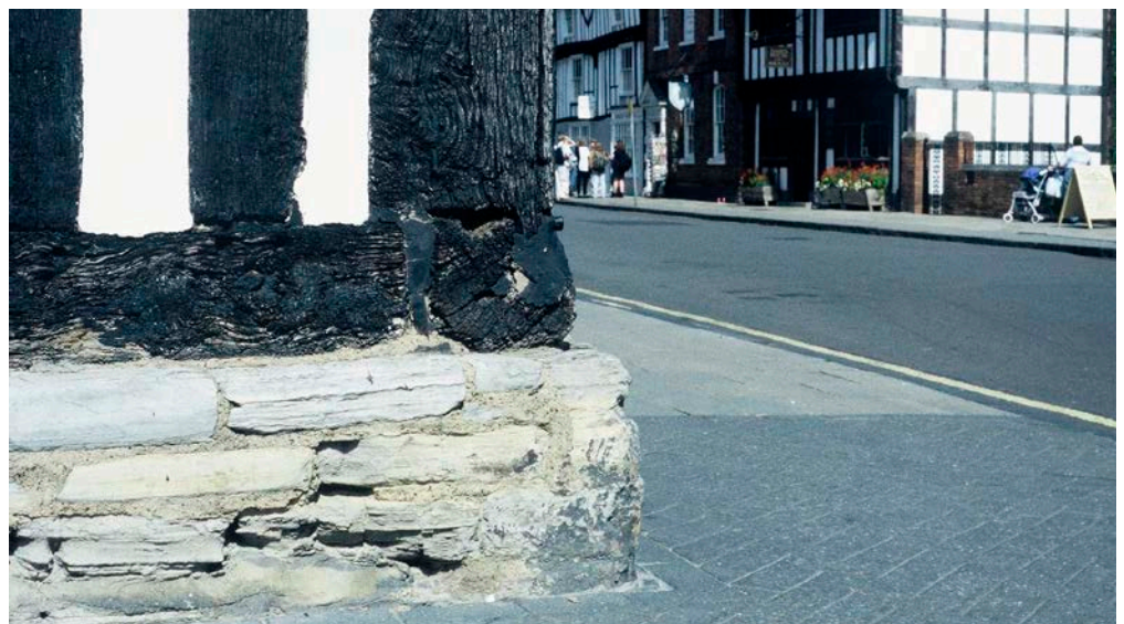
Figure 16: Plinth, timber-framed building. Wilmcot Limestone.
