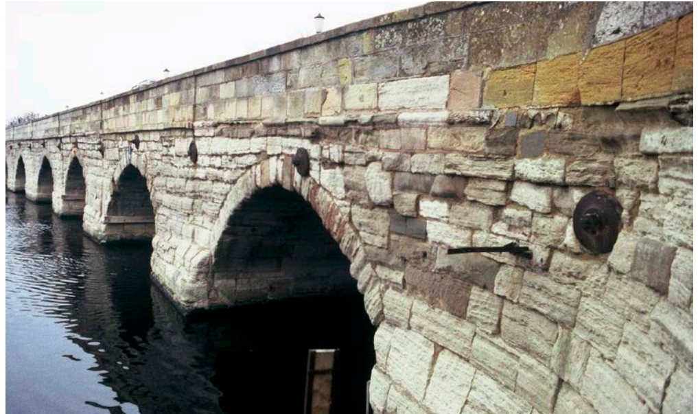
Figure 13: Clopton Bridge. Arden Sandstone.
