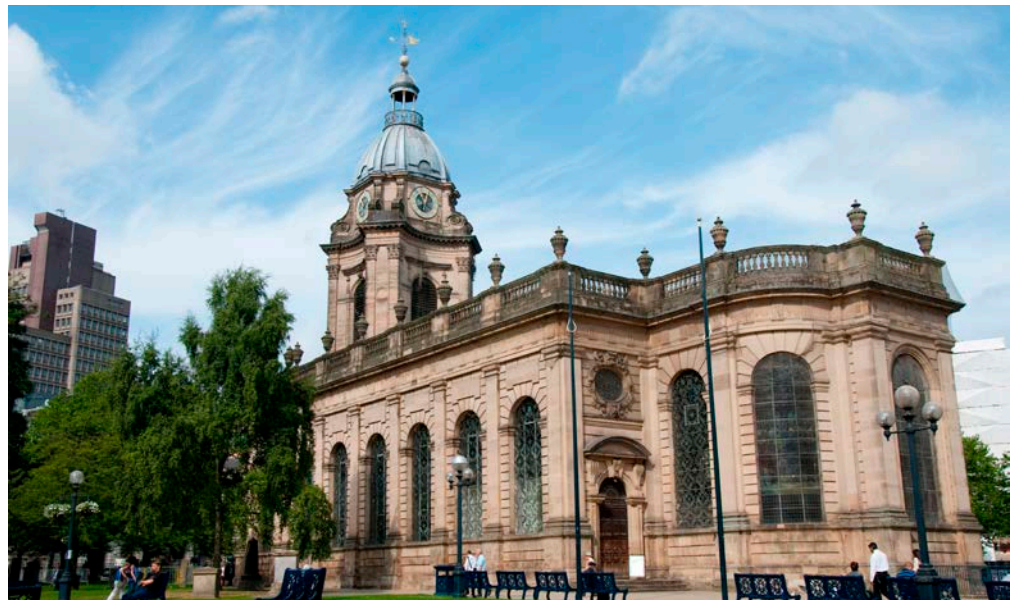
Figure 1: The Cathedral Church of St Philip, Birmingham. Originally constructed of Arden Sandstone but repaired with stones from Derbyshire, Staffordshire and County Durham.
