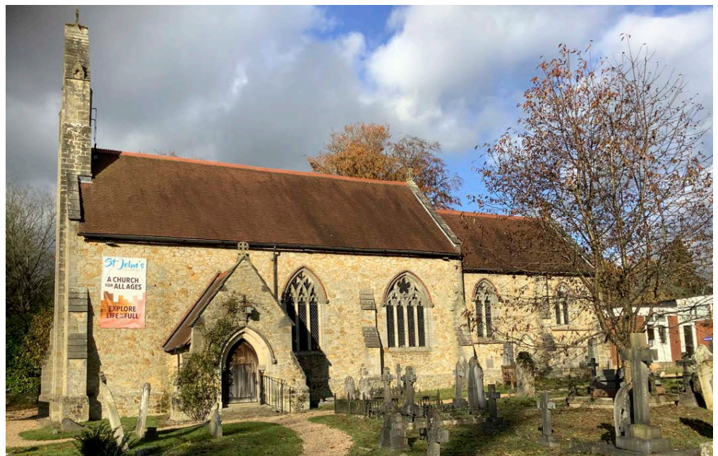
Figure 17: St John the Divine's Church, Felbridge, East Grinstead. Wealden Sandstone.
