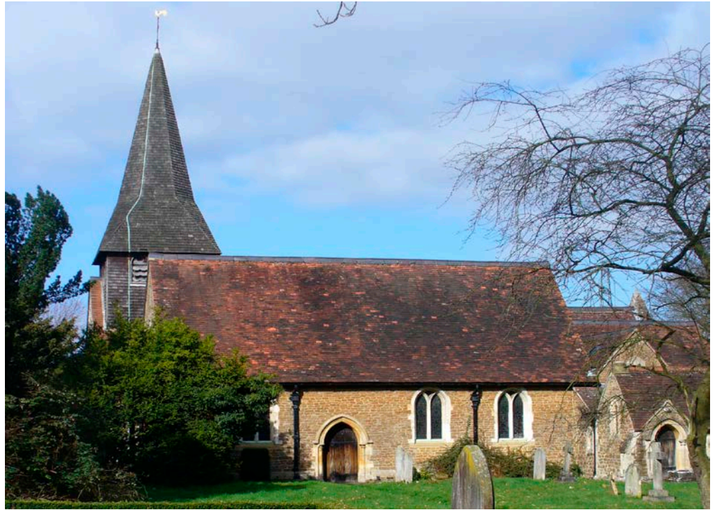
Figure 18: St Mary's Church, Byfleet. Bargate Stone, ironpan conglomerate and flint.
