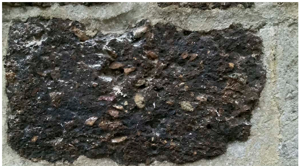
Figure 48: Church of St Nicolas, Cranleigh. Ironpan conglomerate.
