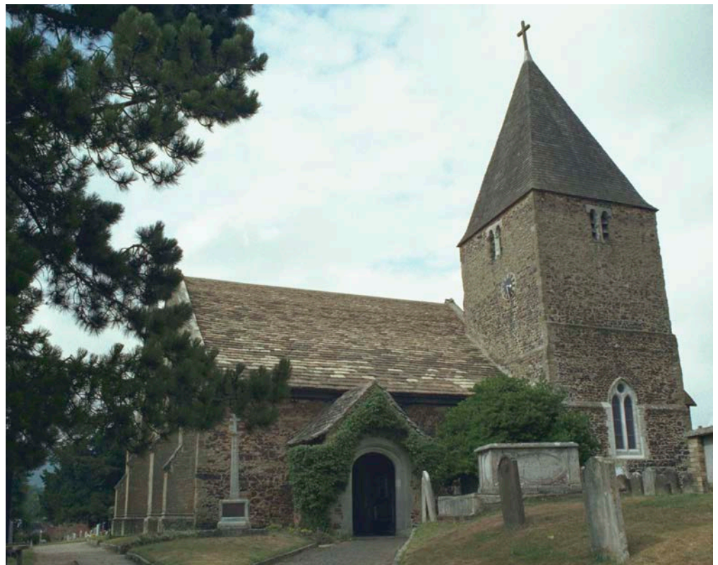
Figure 34: St Peter's Church, Limpsfield. Ironstone rubblestone; Horsham Stone slate nave roof.
