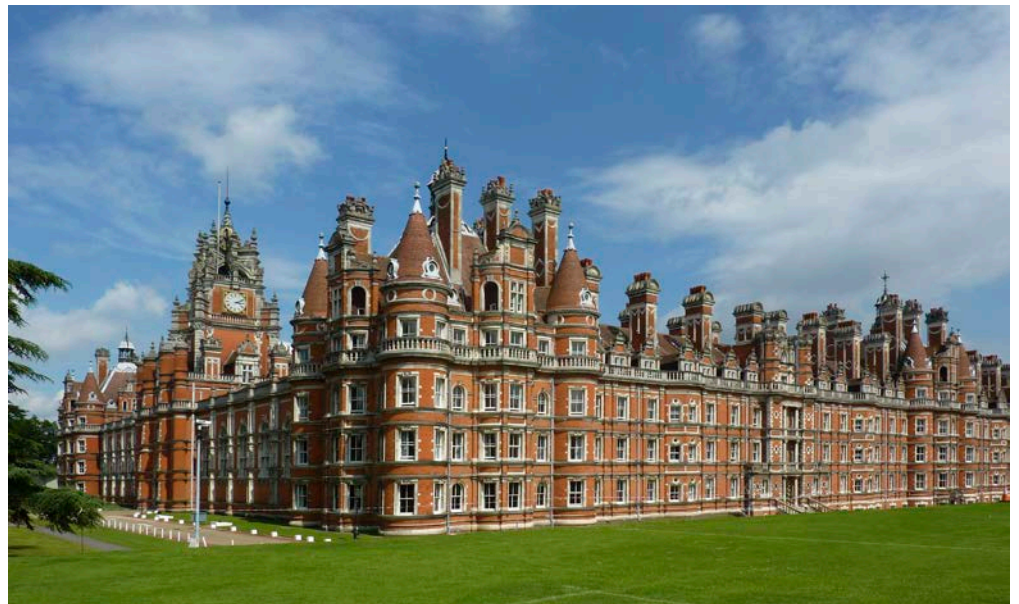
Figure 20: Royal Holloway College, Egham. Brick with Portland Stone dressings and banding.
