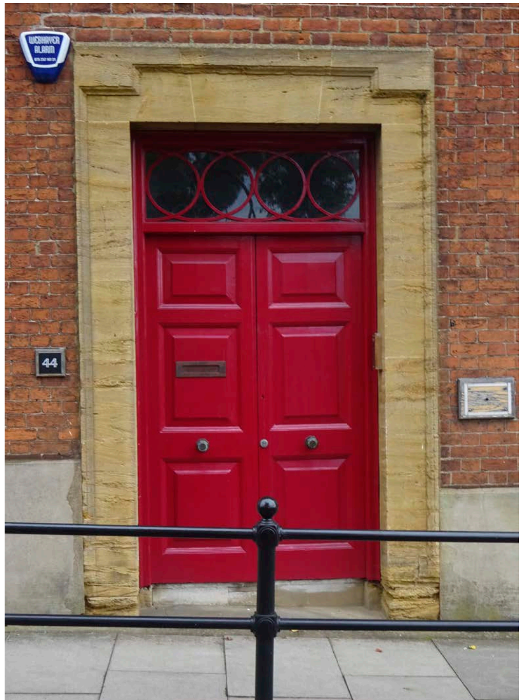
Figure 64: Door surround, 44 Quarry Street, Guildford. Ham Hill Stone.
