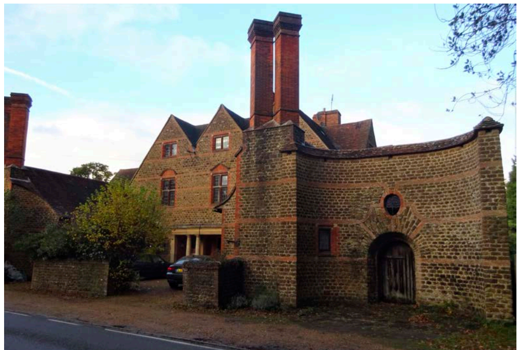
Figure 6: Tigbourne Court, Wormley. Bargate Stone with brick quoins and horizontal tile bands.
