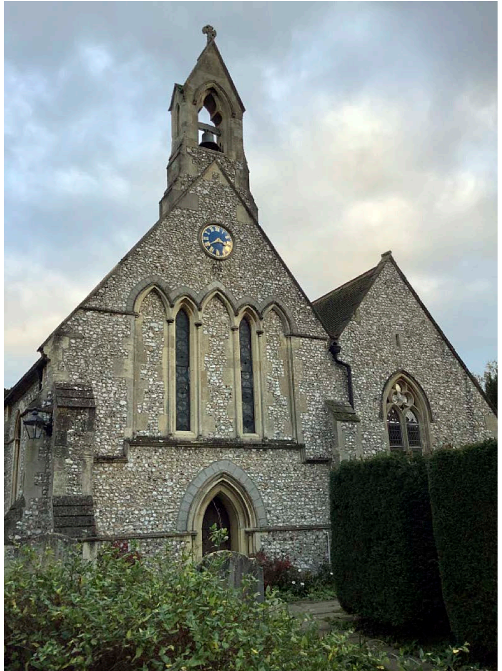
Figure 19: Church of St Mary Magdalen, Ripley. Chancel built in ironpan conglomerate with a Caen stone string course. Chancel built in flint.
