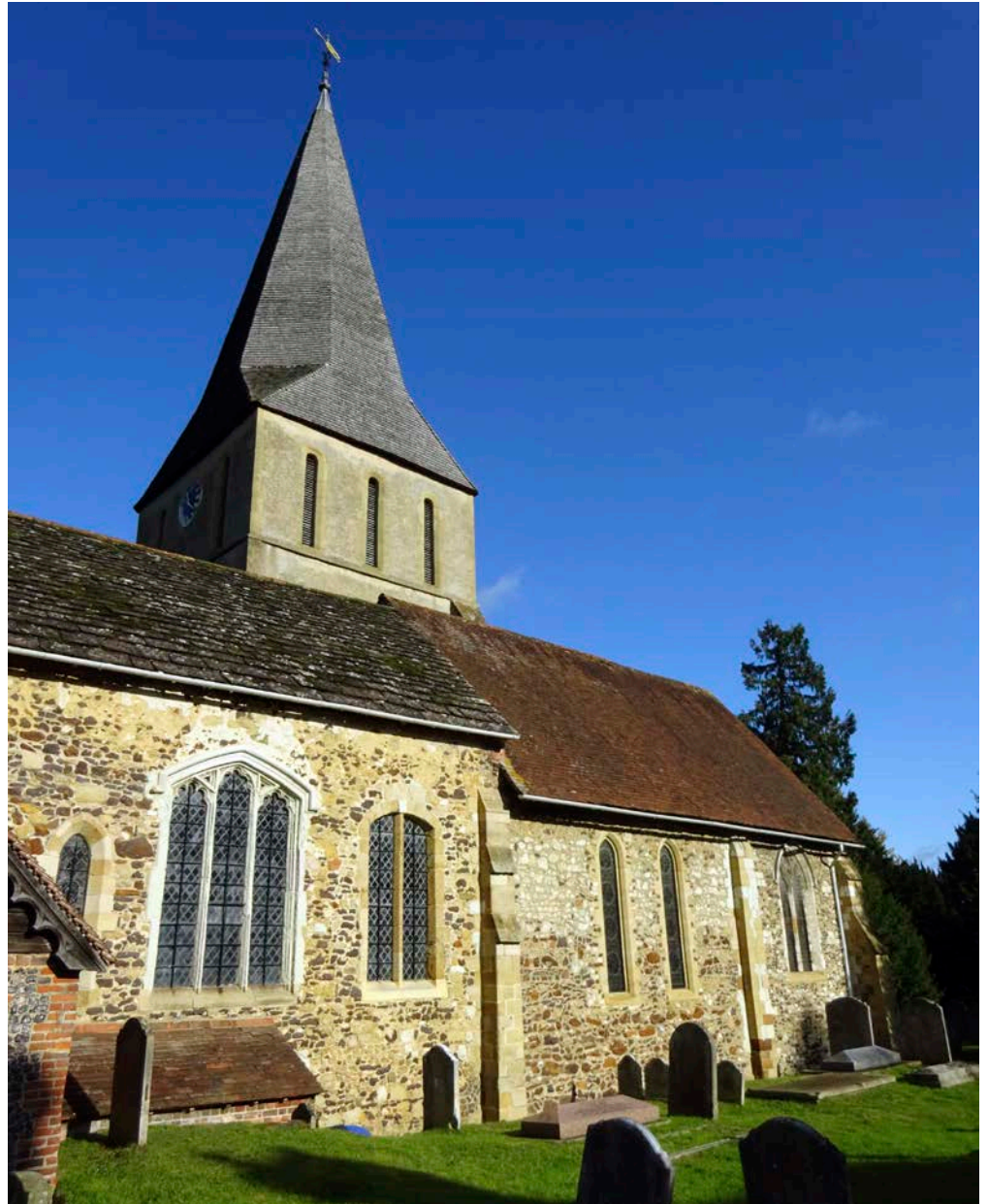
Figure 13: Church of St James, Shere. Carstone, ironpan conglomerate, Quaternary Flint, Caen Stone and Lincolnshire limestone.
