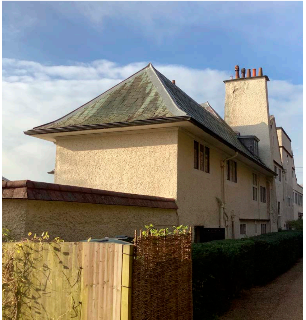
Figure 78: Greyfriars, Wanborough. Westmorland Slate roof.
