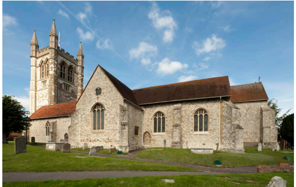
Figure 15: St Andrew's Church, Farnham. Chalk rubble; tower of chalk with Upper Greensand Sandstone and Hollington Stone.
