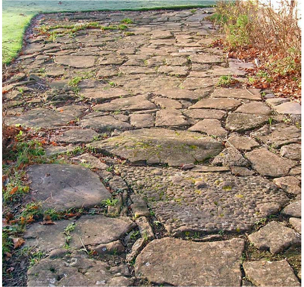
Figure 70: Paving slabs, Dormer Cottage, Stan Hill, Charlwood. Horsham Stone.
