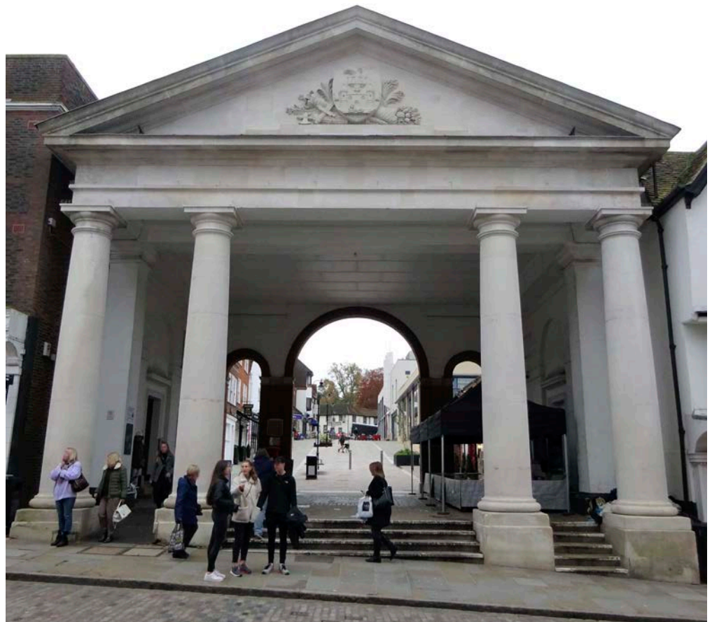
Figure 68: Tunsgate Arch, High Street, Guildford. Portland Stone.
