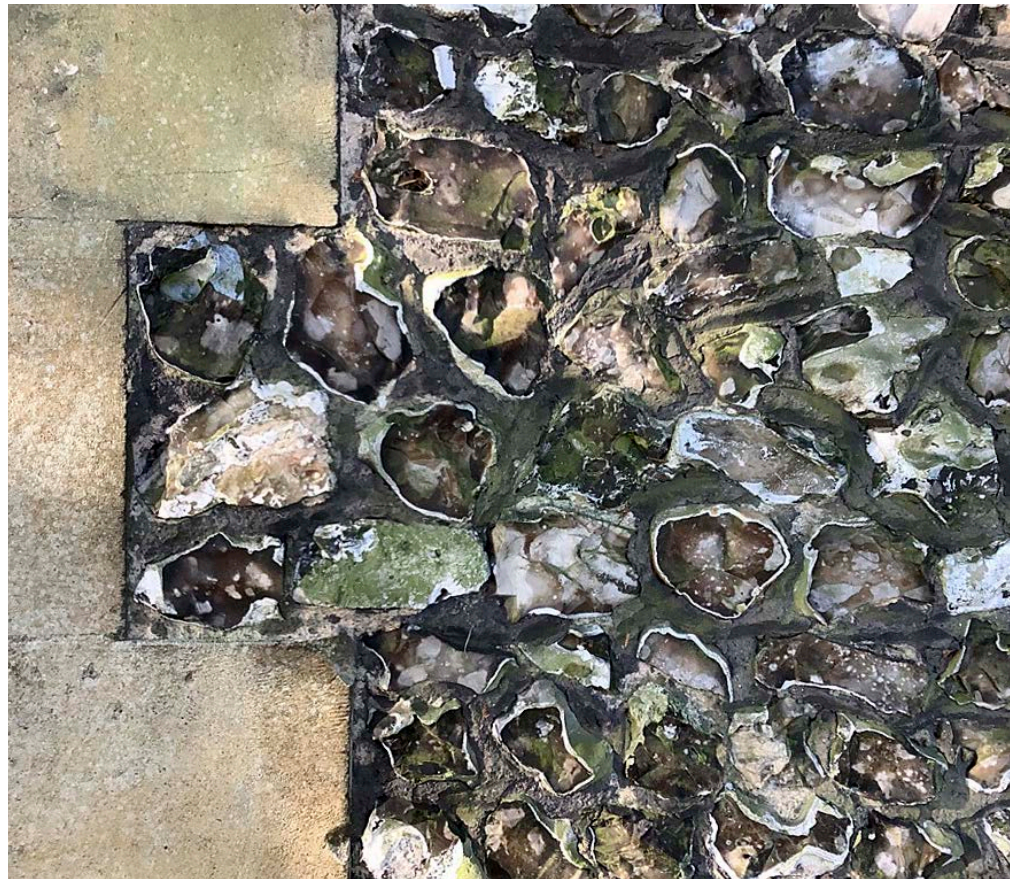
Figure 56: St Nicholas and St Mary Church, Leatherhead. Quaternary Flint and Lincolnshire limestone.
