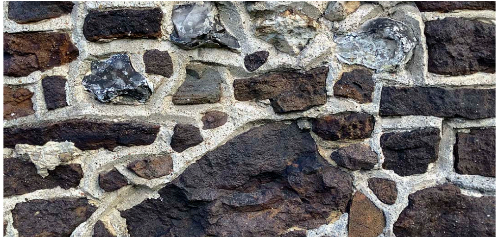
Figure 35: Church of St Mary the Virgin, Buckland. Ironstone blocks.
