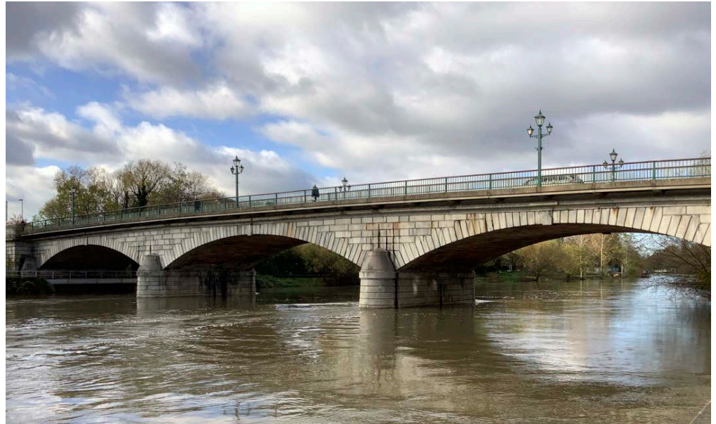
Figure 75: Staines Bridge, Staines. Ashlar granite blocks and corbels.
