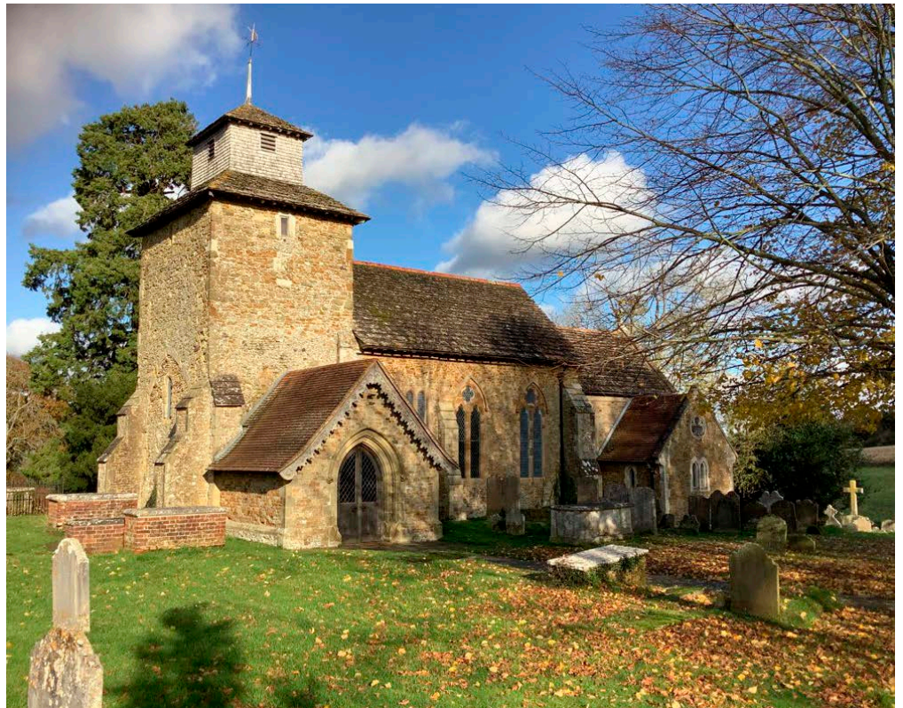
Figure 71: St John the Evangelist Church, Wotton. Bargate Stone with Firestone and Bath Stone dressings. Horsham Stone slate roof.
