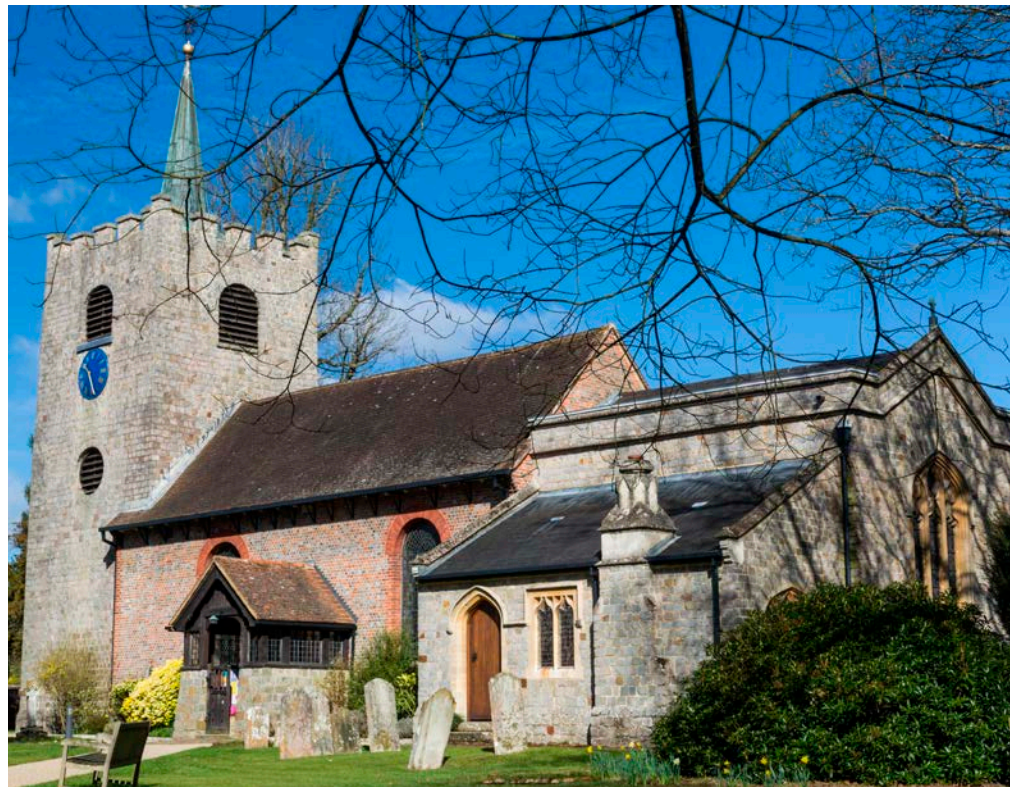
Figure 51: Church of St Michael and All Angels, Pirbright. Sarsen stone with Bath Stone and brick dressings.
