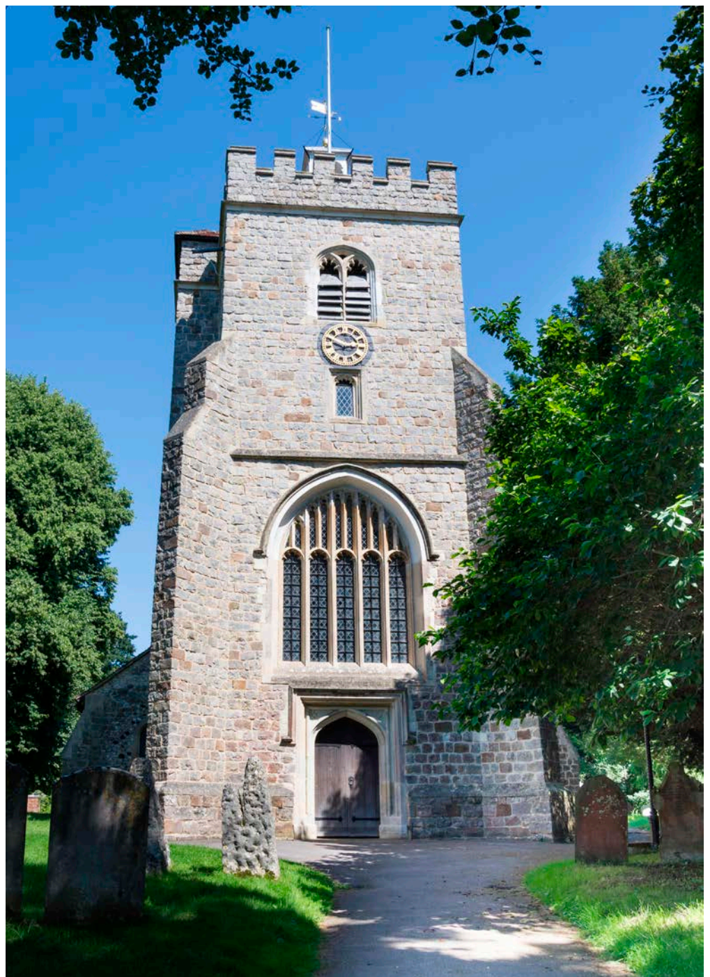
Figure 53: Tower, Church of St Mary the Virgin, Worplesdon. Sarsen stone.
