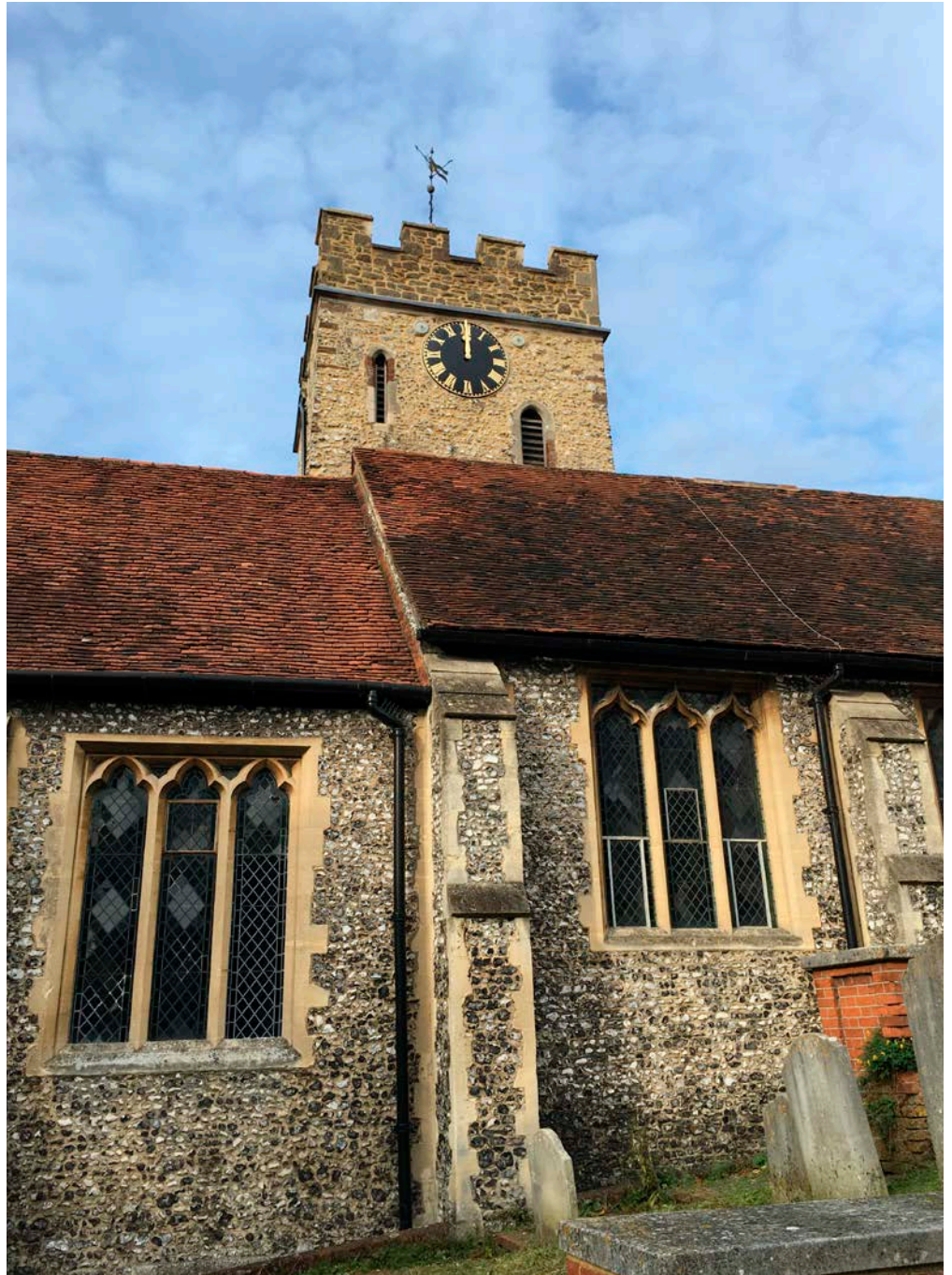
Figure 59: St Mary's Church, Guildford. Flint and chalk.
