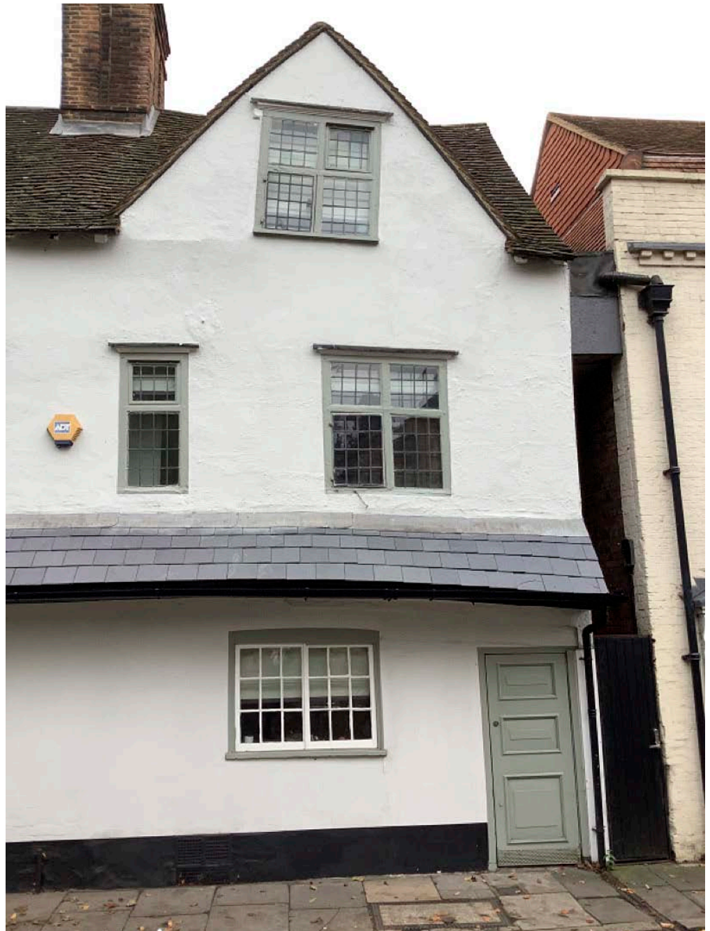
Figure 77: 19 Quarry Street, Guildford. Welsh Slate porch roof.
