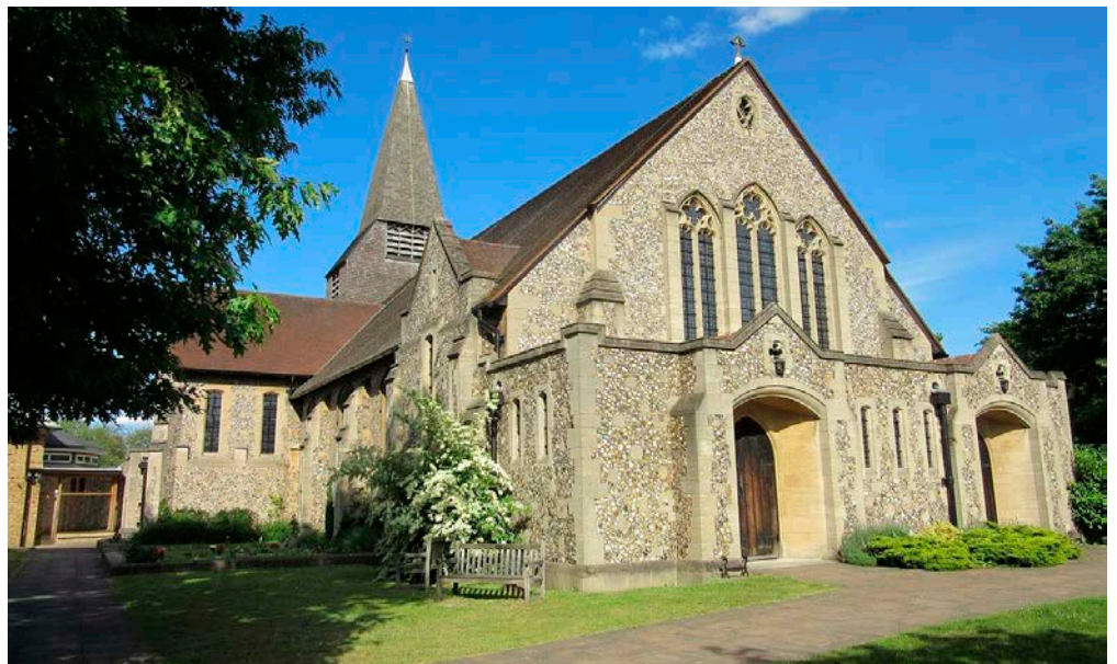
Figure 54: Church of St John the Baptist, West Byfleet. Quaternary Flint and chert with blocks and dressings of Lincolnshire limestone and Bath Stone.
