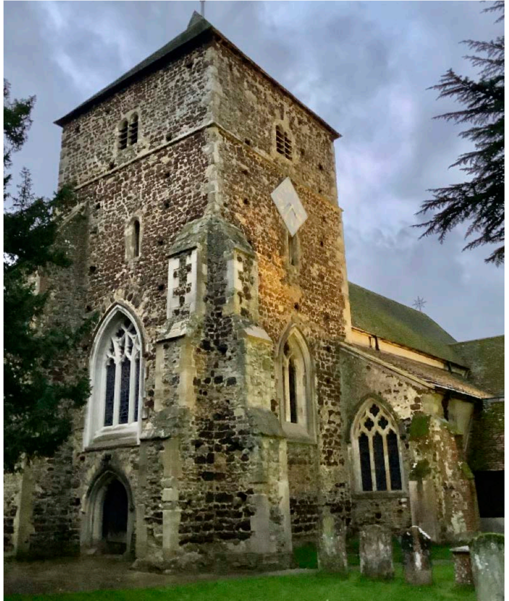
Figure 47: Tower, Church of St Nicolas, Cranleigh. Ironpan conglomerate, ironstone and Bargate Stone with dressings of chalk, Bath Stone and Lincolnshire limestone.
