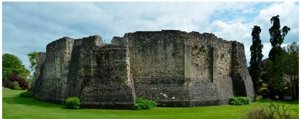
Figure 21: Curtain wall and keep, Farnham Castle. Chalk and Upper Greensand Sandstone.
