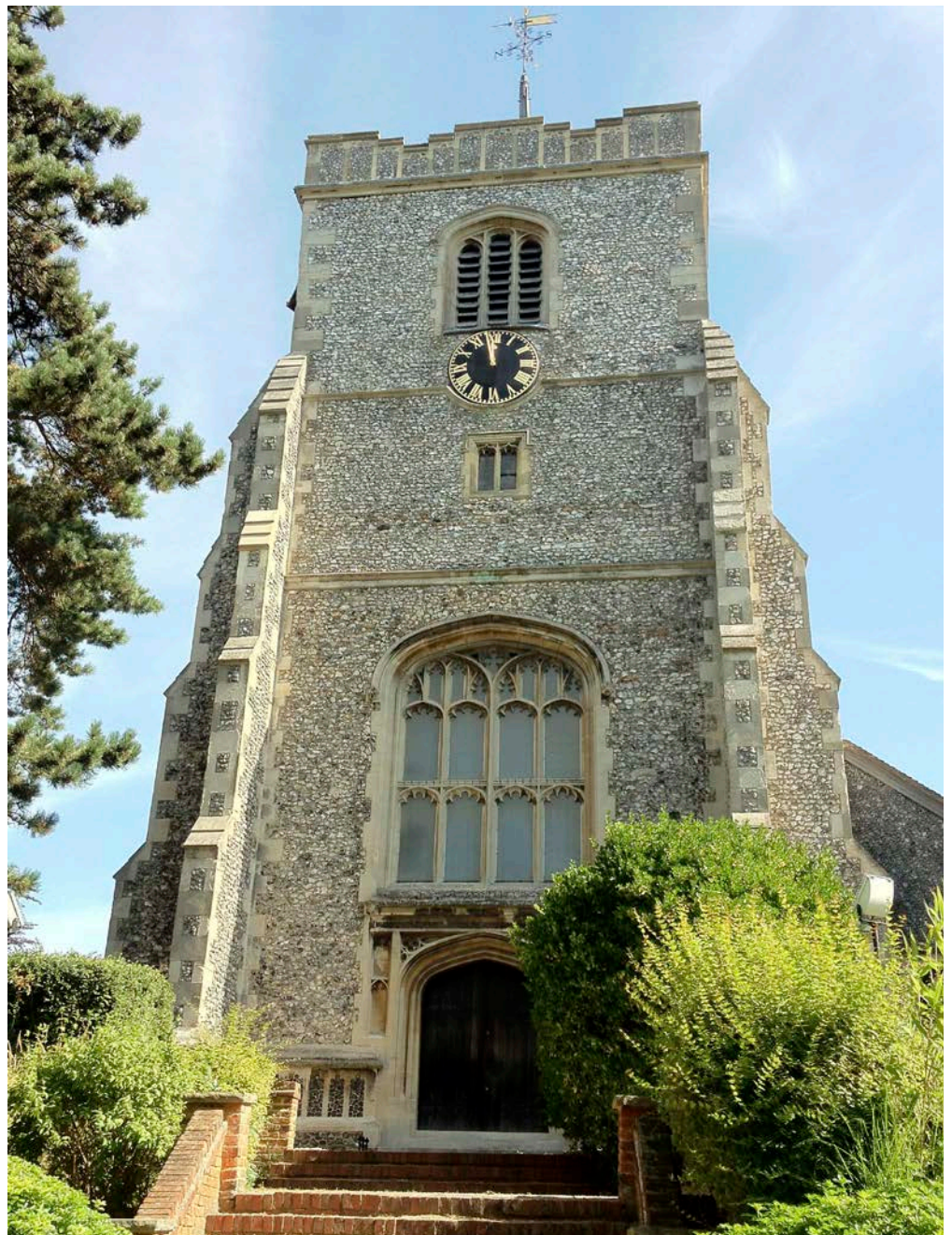
Figure 65: St Nicholas and St Mary's Church, Leatherhead. Quaternary Flint with dressings of Lincolnshire limestone; the north transept has a Horsham Stone slate roof.
