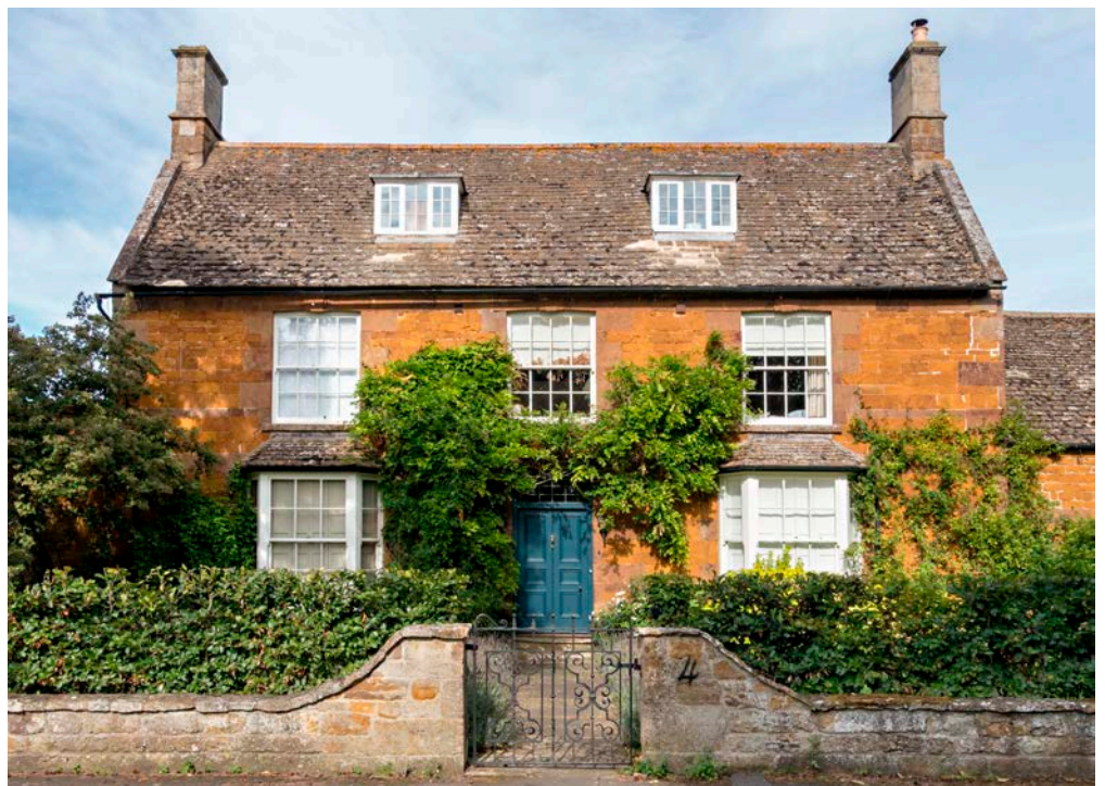
Figure 6: Bell House, Lyddington. Collyweston Stone slate roof and Northampton Stone ashlar.
