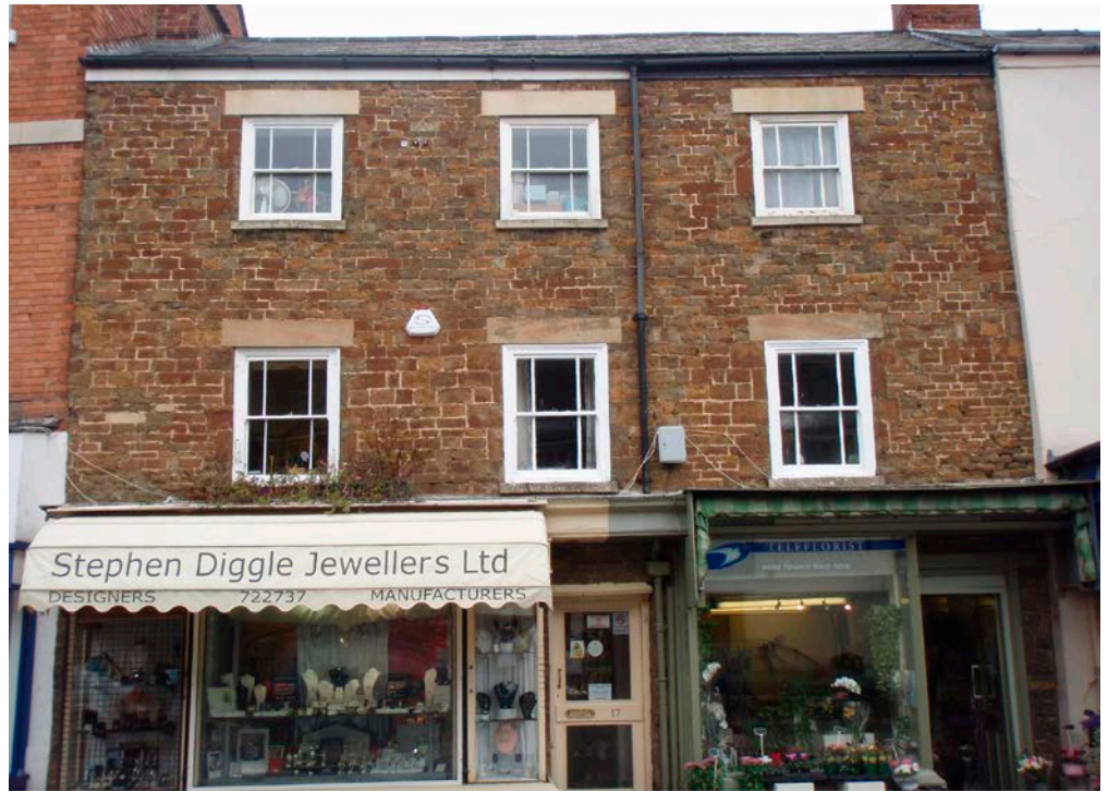
Figure 2: High Street, Oakham. Northampton Stone.
