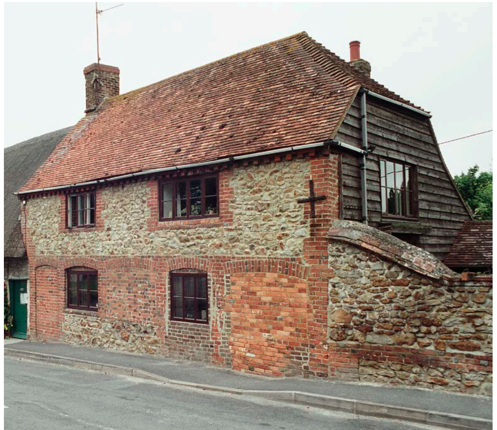
Figure 15: Old Forge Cottage, High Street, Ashbury, Vale of White Horse. Uncoursed Sarsen Stone rubble with brick quoins and dressings.
