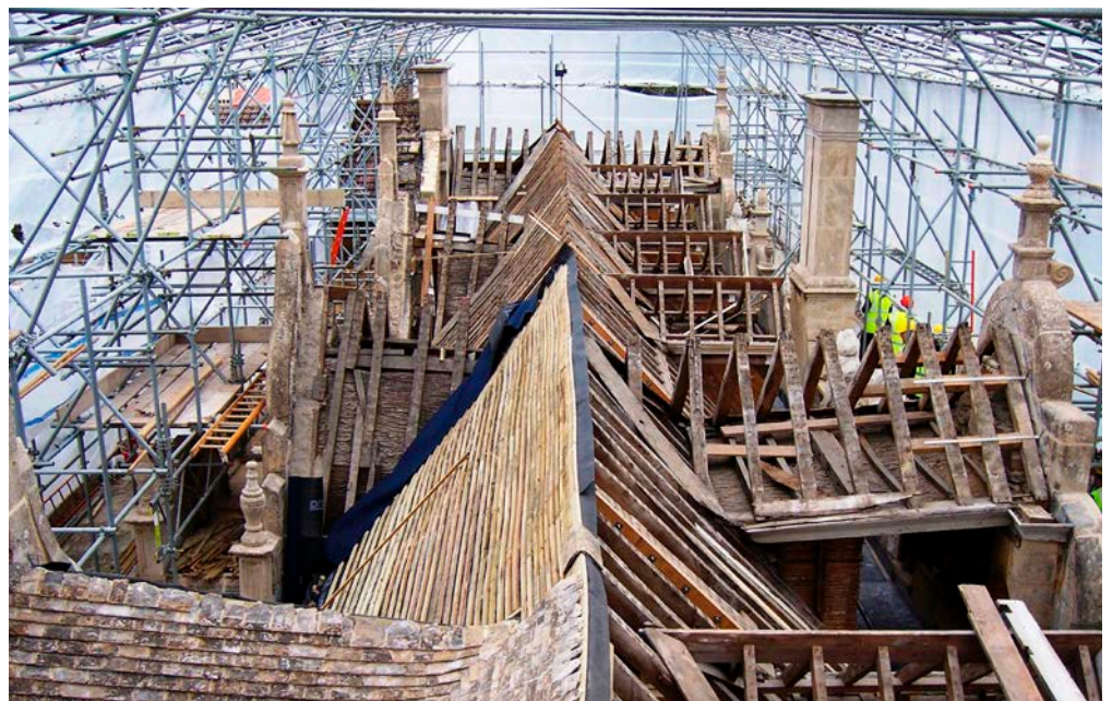
Figure 17: Restoration work, Apethorpe Palace, Apethorpe. Collyweston Stone slate.
