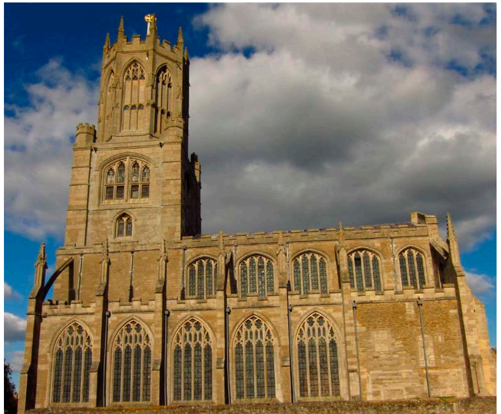
Figure 18: Church of St Mary and All Saints, Fotheringhay. Upper Lincolnshire Limestone with Stanion-like Stone walls and buttresses. King's Cliffe Stone in the parapet and north porch.
