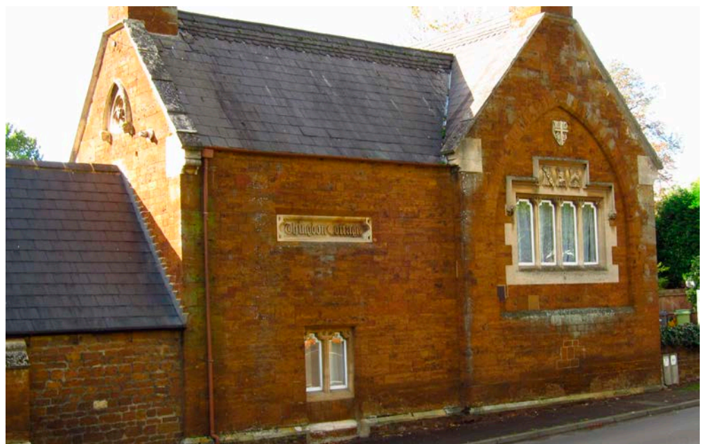
Figure 6: Abbingdon Cottage, Finedon. Finedon Stone and Weldon Stone.
