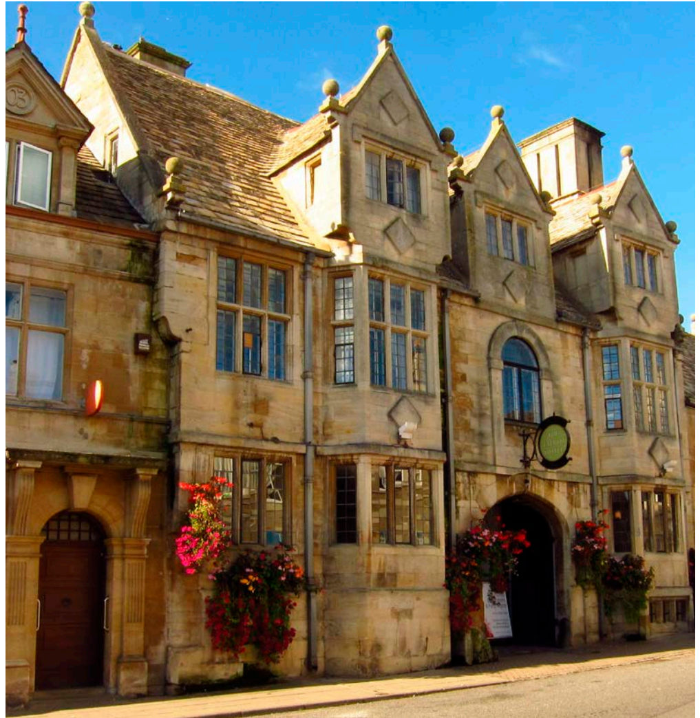
Figure 20: Talbot Inn, New Street, Oundle. Weldon Stone with Lincolnshire Limestone tracery and finials.
