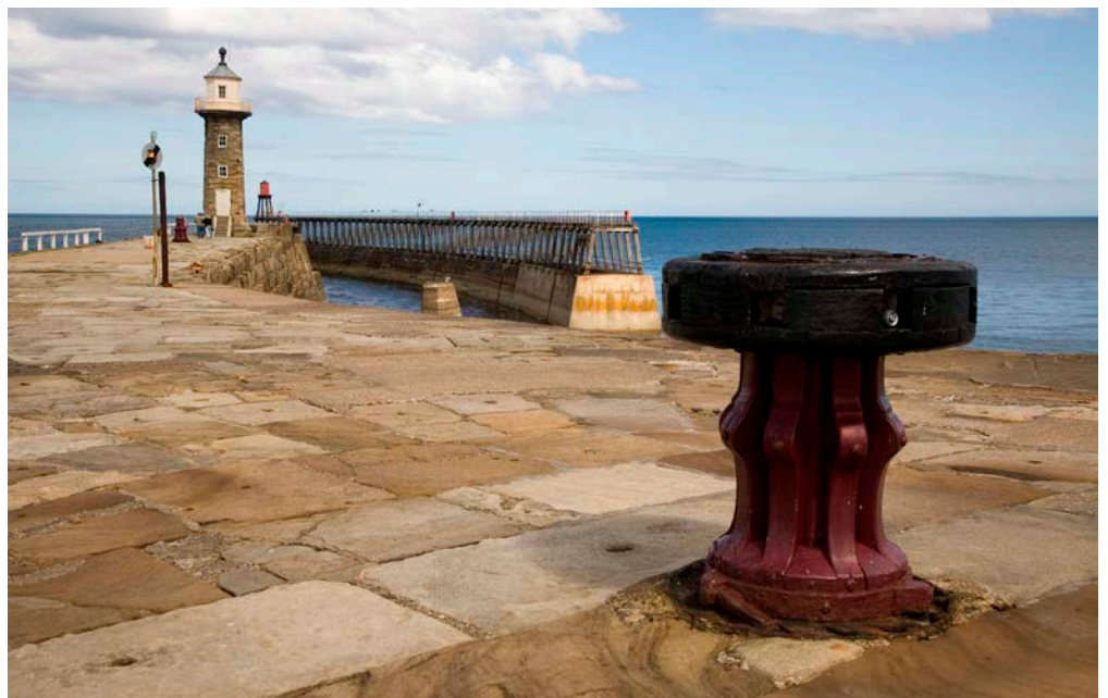
Figure 10: Whitby harbour flagstones. Moor Grit Member Sandstone.
