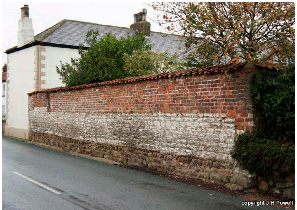
Figure 23: Wall, Bempton. Sandstone and quartzite boulders with higher courses of chalk and red brick.
