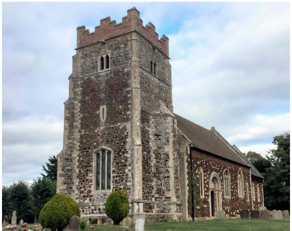
Figure 7: Church of St Mary the Virgin, Wimbotsham. Cinderstone and Big Carr with Lincolnshire Limestone and Totternhoe Stone dressings.
