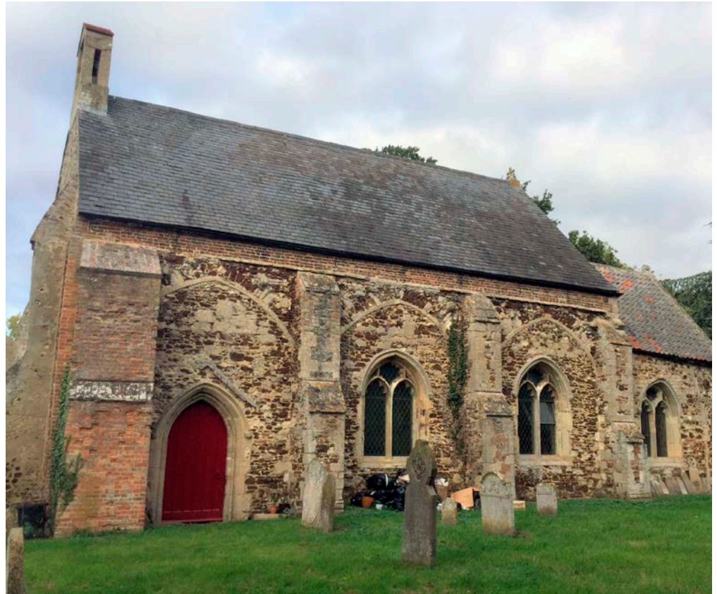
Figure 49: St Mary's Church, Fordham. Lincolnshire Limestone and ironbound sandstone.
