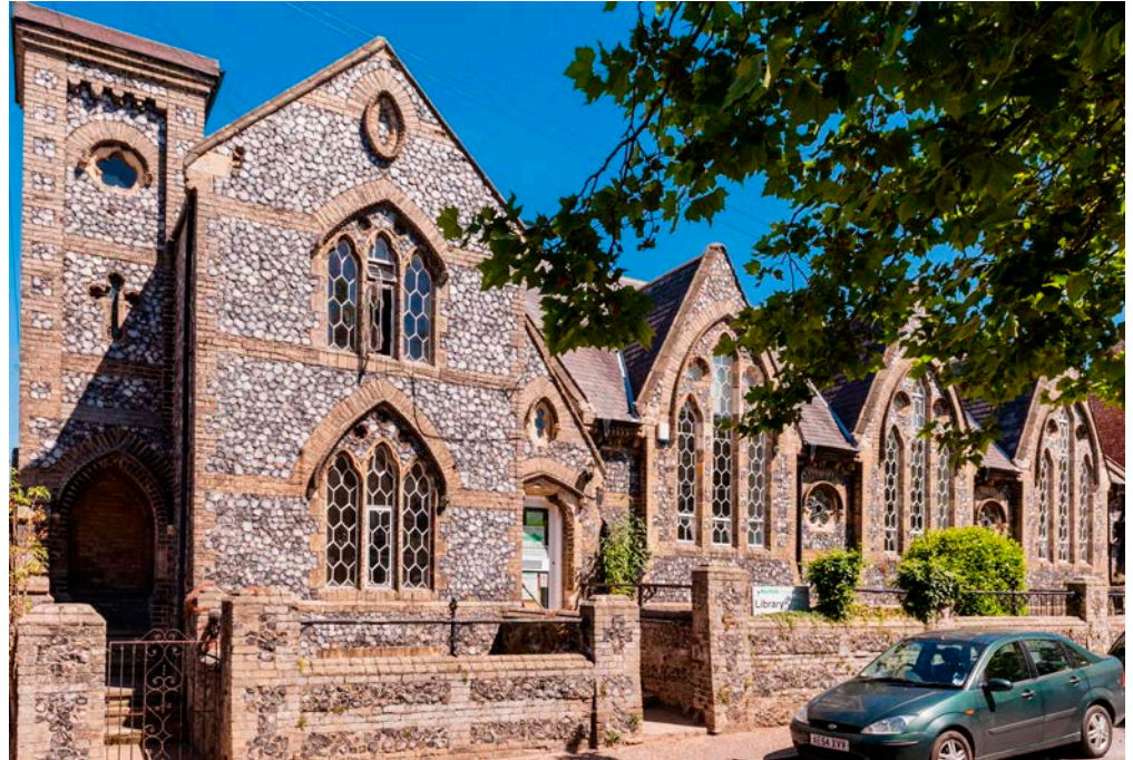
Figure 19: Library, Loddon. Quaternary Flint with brick and limestone dressings.
