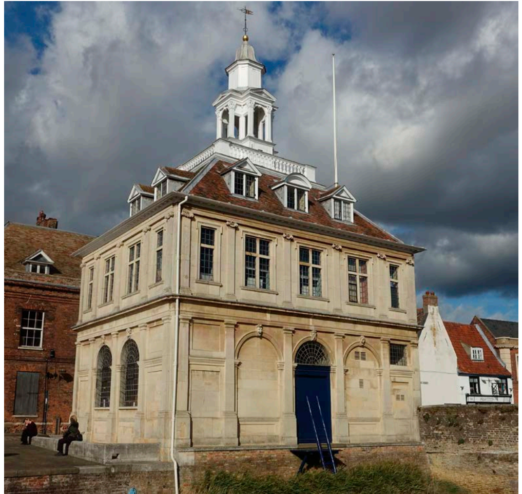
Figure 68: The Custom House, Purfleet Quay, King's Lynn. Ketton Stone.
