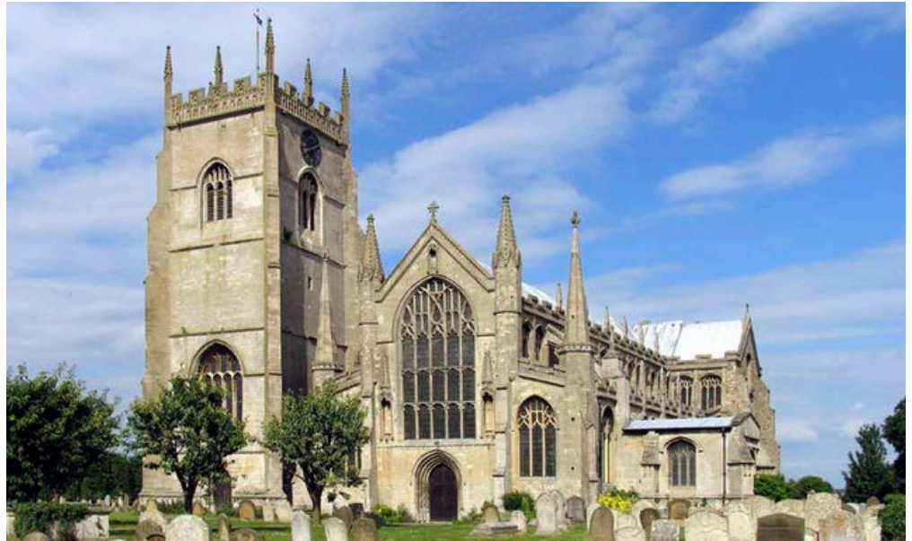
Figure 6: Church of St Clement, Terrington St Clement. Lincolnshire Limestone and Big Carr.
