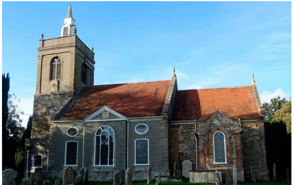
Figure 47: All Saints' Church, North Runcton. Ironbound conglomerate, ironbound sandstone, Cinderstone, carstone and Quaternary Flint.
