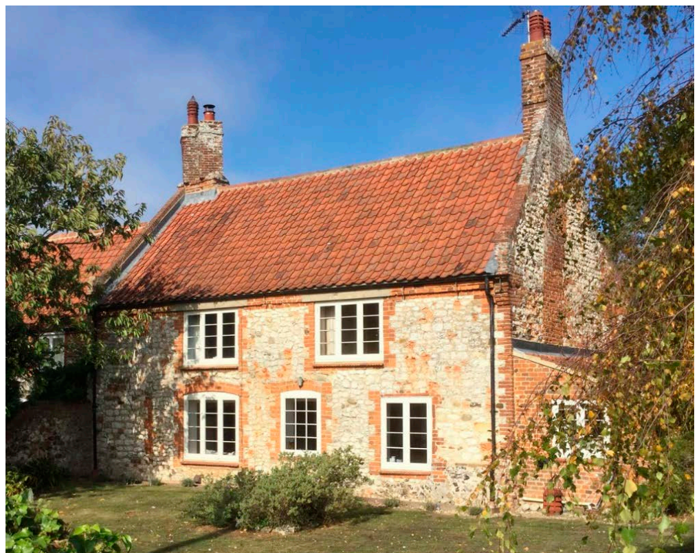
Figure 12: Cottage, Holme-next-the-Sea. Chalk and Red Chalk with flint, carstone and brick dressing.
