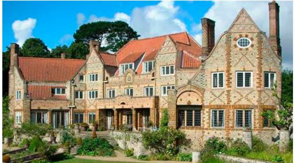
Figure 4: Voewood, Kelling, Holt. Quaternary Flint facing and Big Carr dressings and details.
