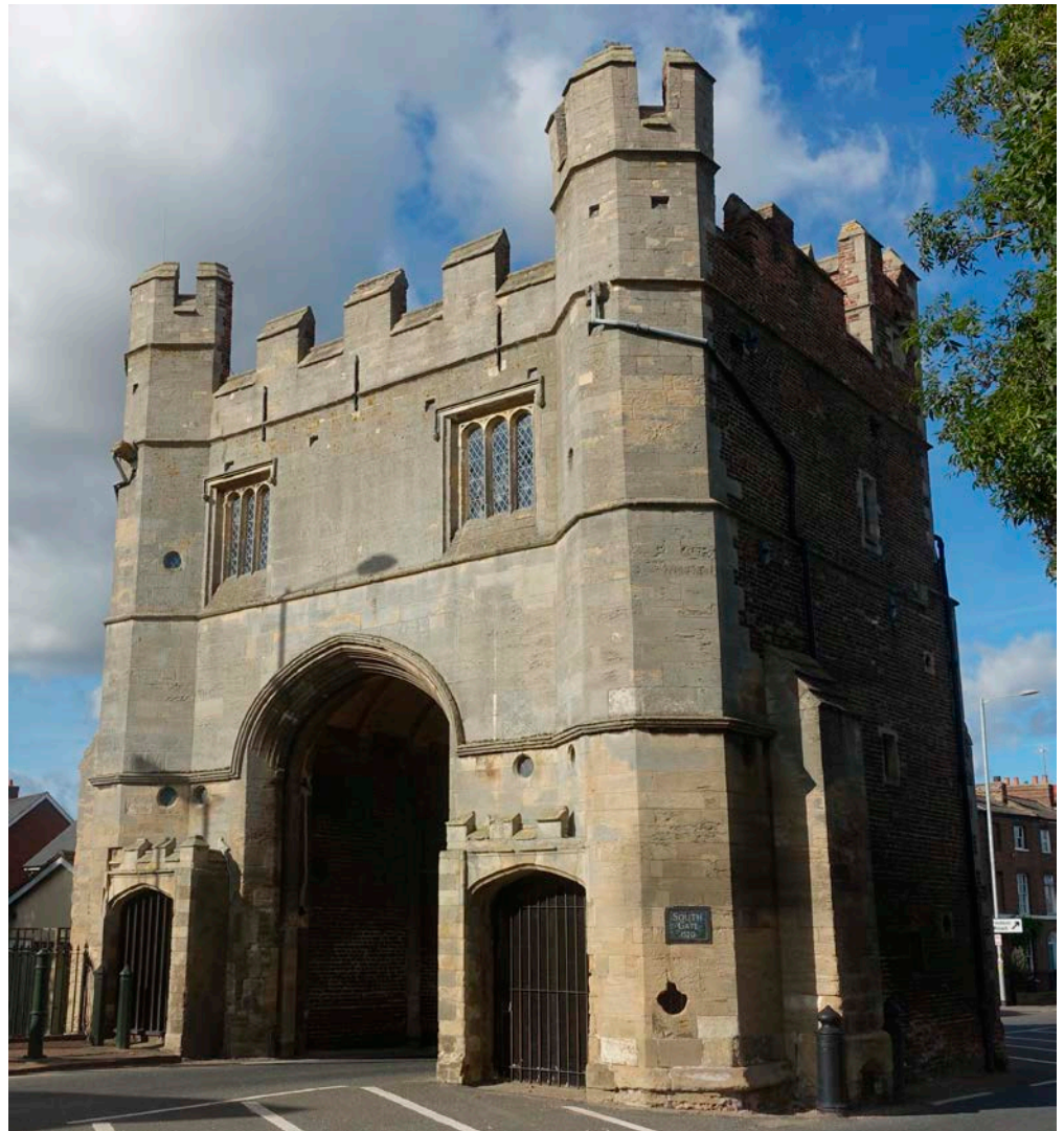
Figure 67: South Gate, King's Lynn. Restored with Lincolnshire limestone. Originally built with Barnack Stone.
