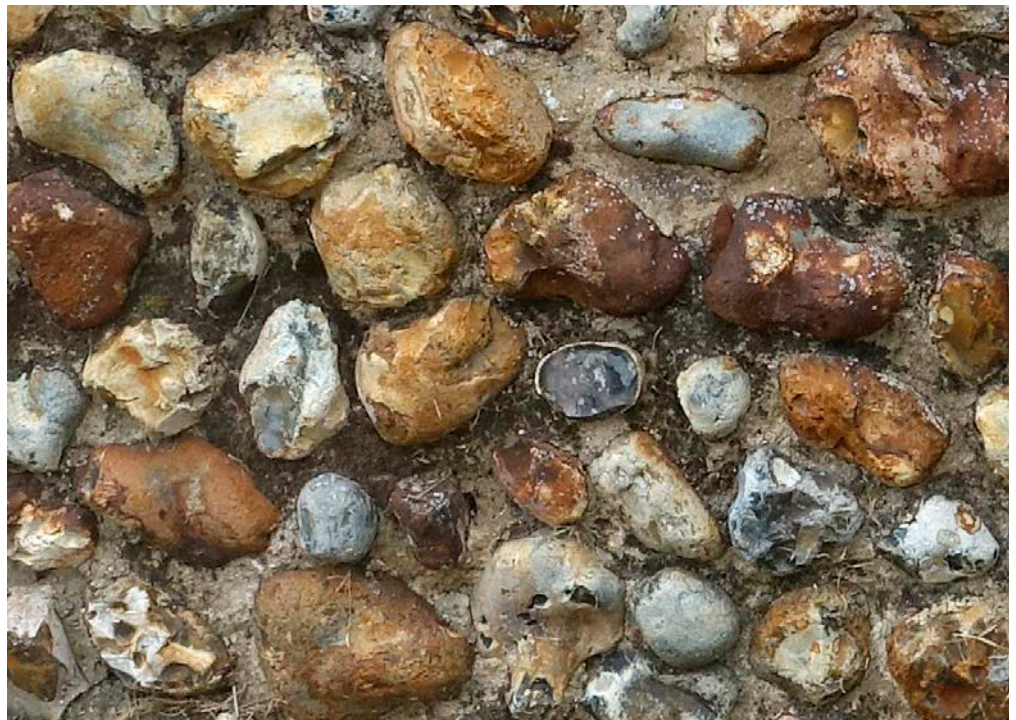
Figure 52: Churchyard wall, Church of All Saints, Shipdham. Chert pebbles and cobbles with some Quaternary Flint pebbles.
