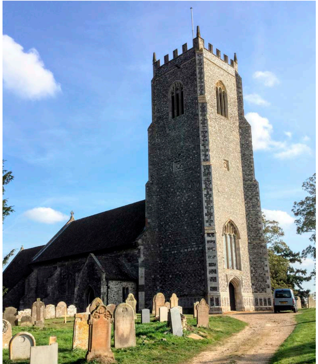
Figure 18: Church of St John the Baptist, Reedham. Leziate Quartzite, Quaternary Flint, Chalky Hardpan, Ironpan and Lincolnshire Limestone.
