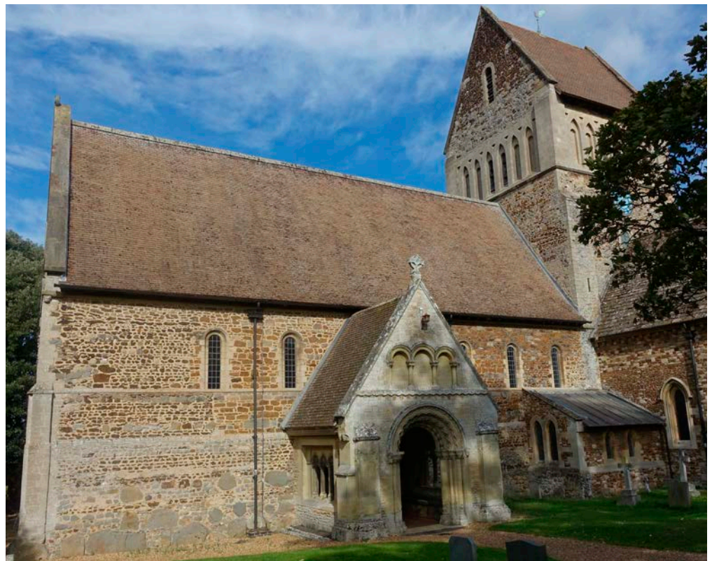
Figure 26: St Lawrence's Church, Castle Rising. Carstone and Leziate Quartzite with Lincolnshire Limestone dressings.
