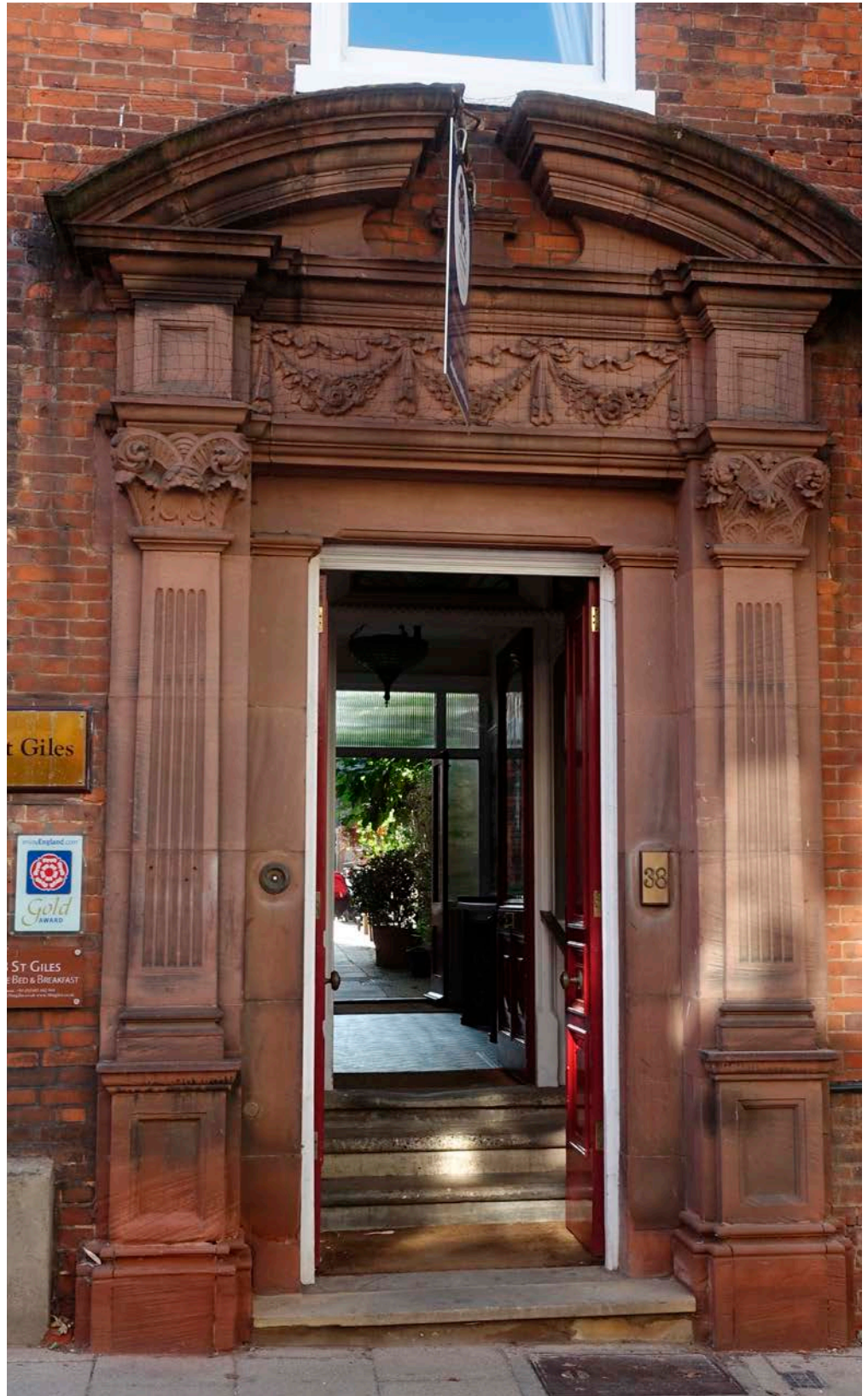
Figure 65: Doorway, 38 St Giles Street, Norwich. Mansfield Red Stone.
