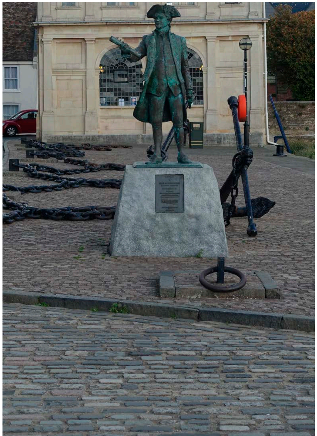
Figure 74: Paving and road setts, Purfleet Quay, King's Lynn. Granite.
