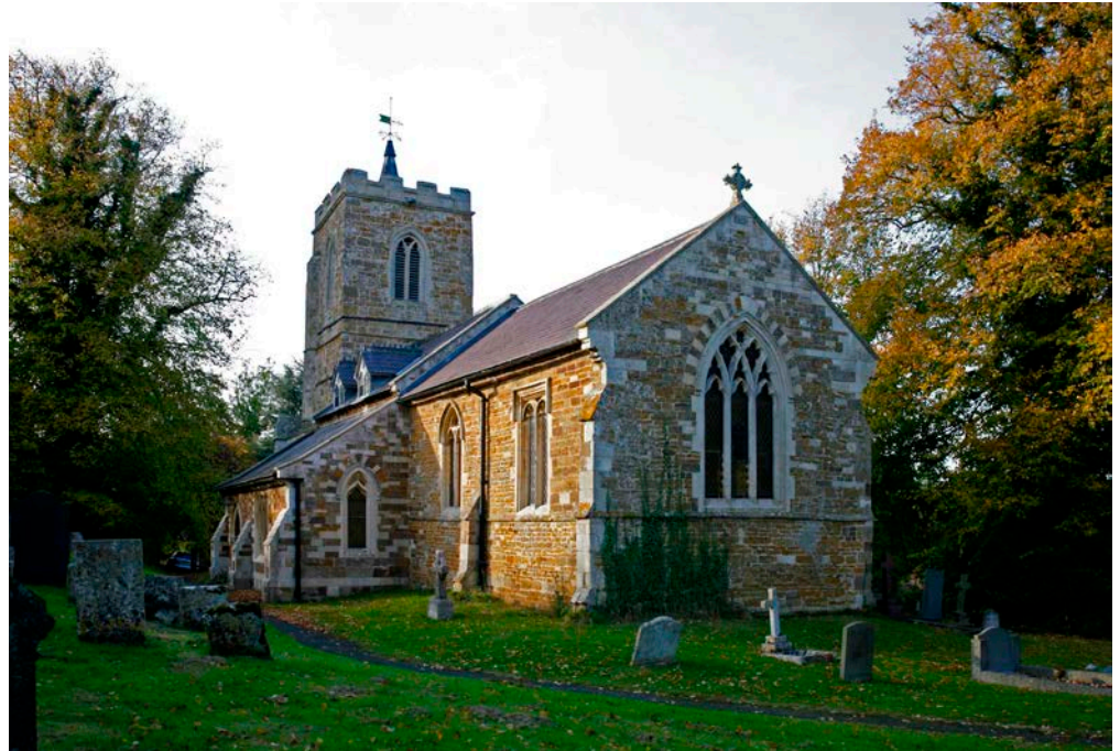
Figure 1: Church of St Peter, Allexton. Northampton Sand, Lincolnshire Limestone dressings and Millstone Grit repairs.
