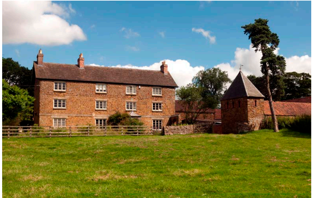
Figure 2: Farm buildings, Wartnaby. Sandrock.
