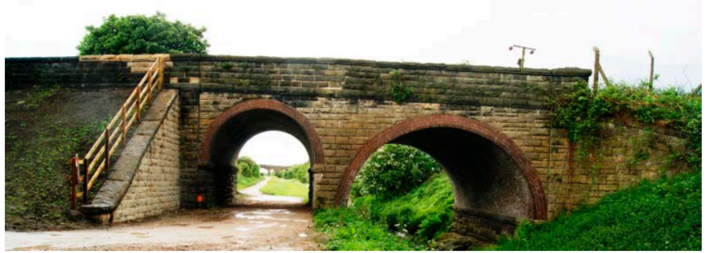
Figure 28: Great Altcar railway bridge. Ormskirk Sandstone.
