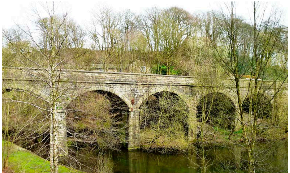
Figure 15: Holcombe Road Viaduct, Haslingden. Fletcher Bank Grit and Rough Rock.
