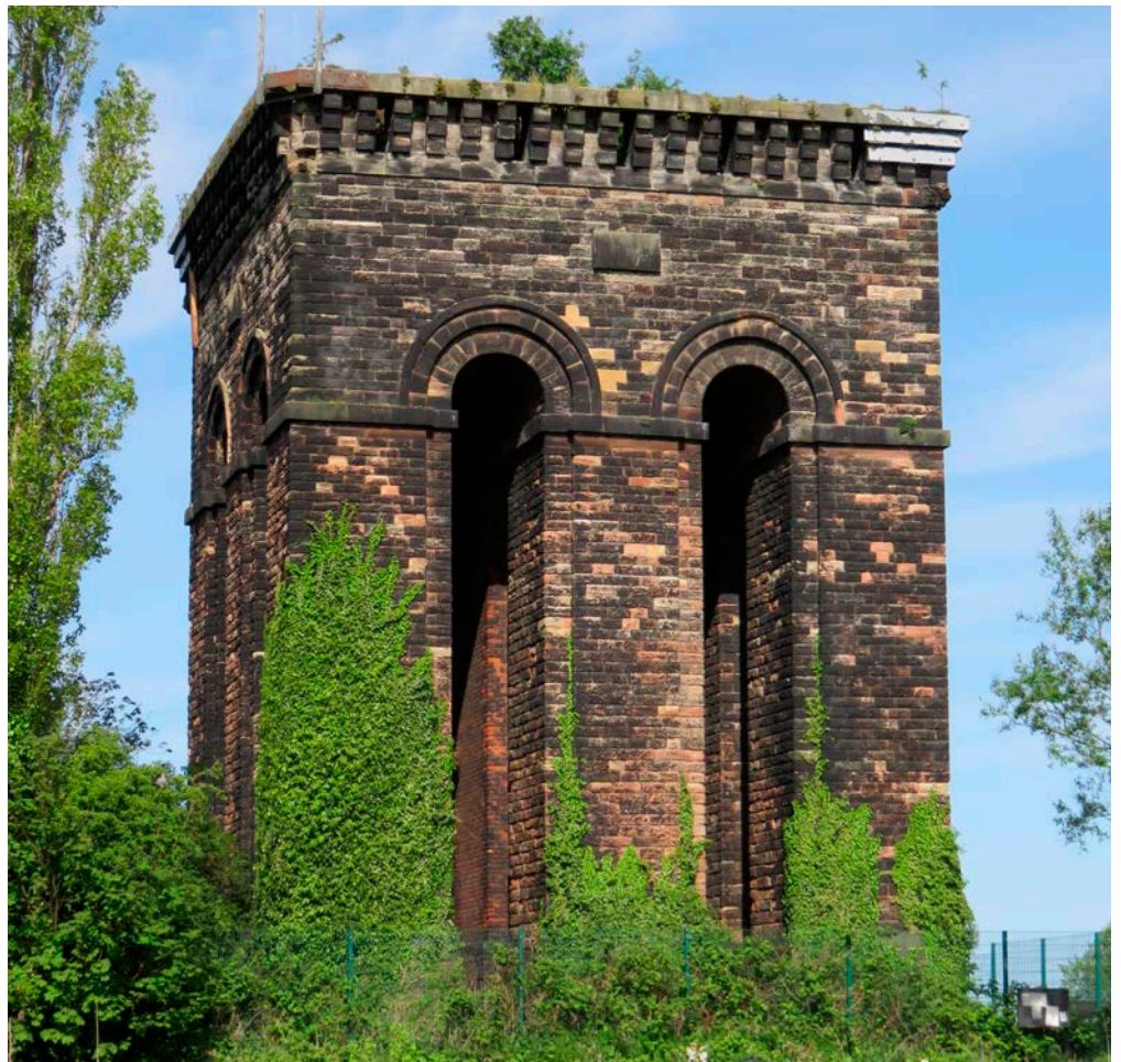
Figure 30: Water Tower, Tower Hill, Ormskirk. Ormskirk Sandstone.
