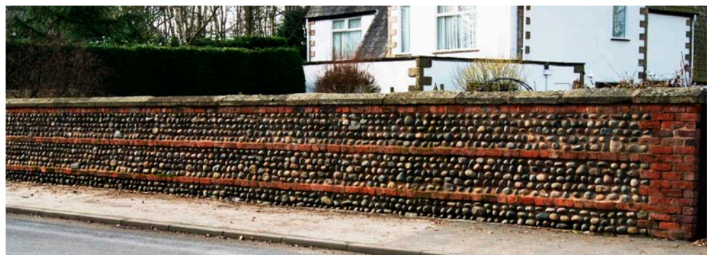
Figure 31: Lytham Hall boundary walls. Cobbles.
