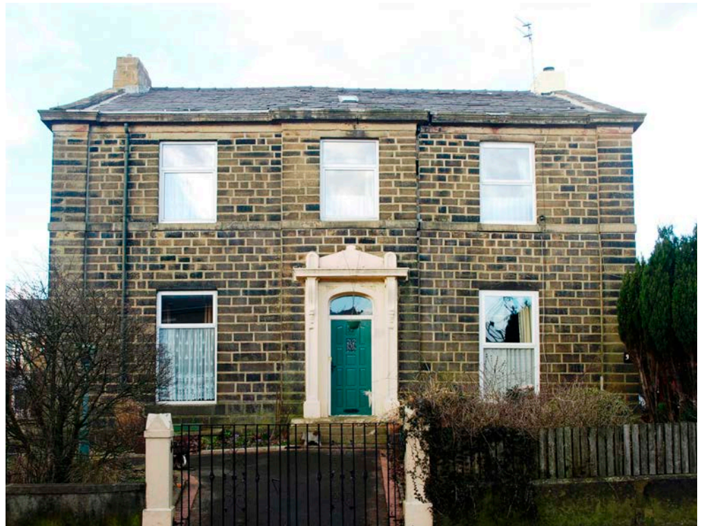
Figure 23: House, Clayton-le-Moors. Old Lawrence Rock.
