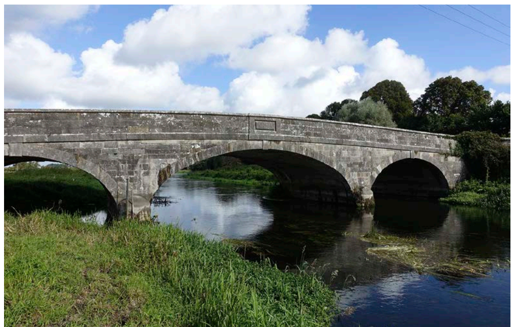
Figure 26: Ibsley Bridge, near Harbridge. Purbeck Stone.
