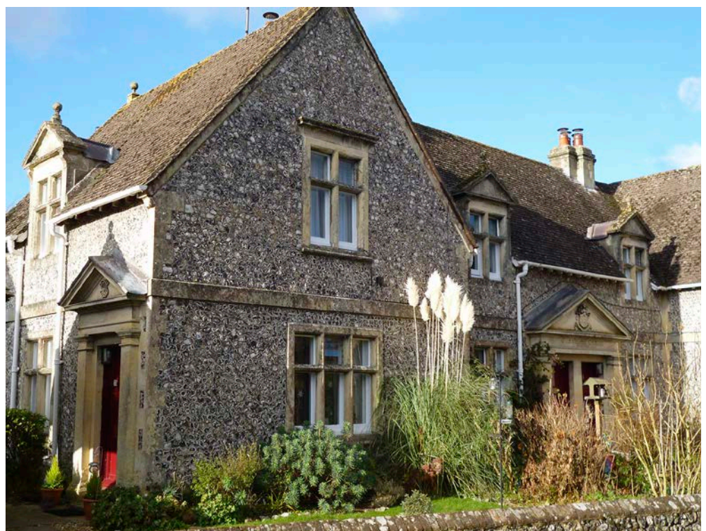
Figure 13: Forbes Almshouses, East Meon. Knapped flint nodules with Bath Stone dressings.
