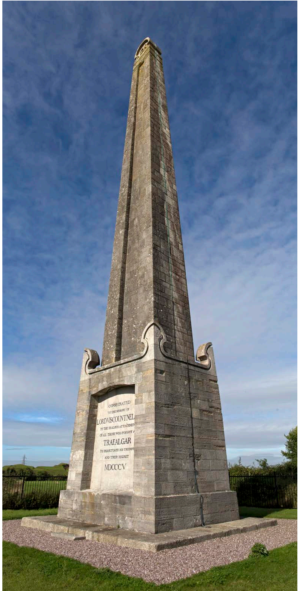
Figure 24: Nelson Monument, Boarhunt. Portland Stone ashlar on a granite base.
