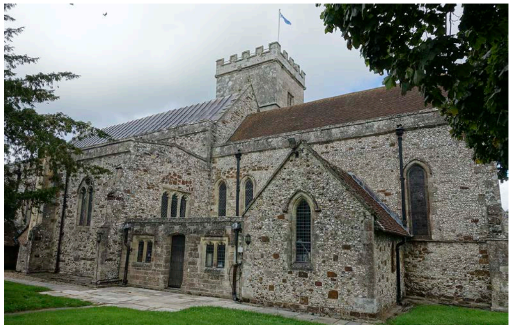
Figure 6: Church of St Mary, Fordingbridge. Flint nodules with blocks of Malmstone, Reading Beds Sandstone and ferricrete.
