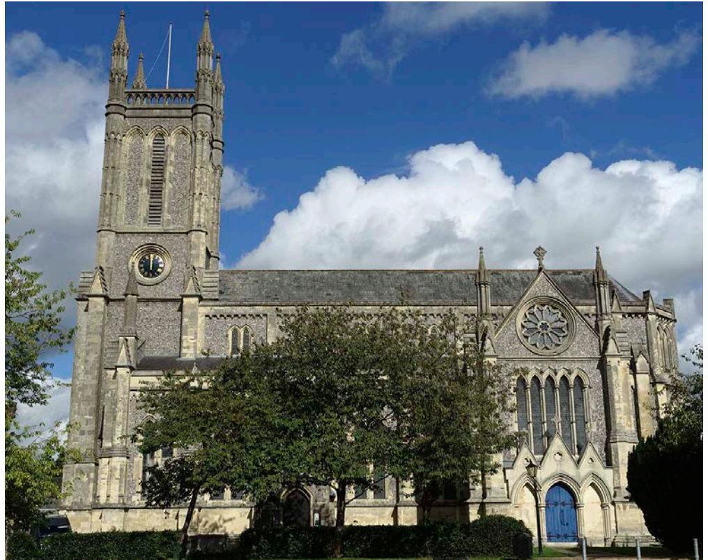
Figure 21: Church of St Mary, Andover. Knapped flint walls and Caen Stone dressings.
