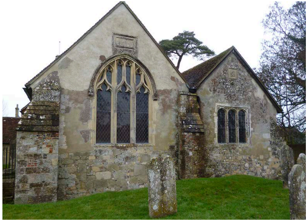
Figure 30: Church of St James, Southwick. Green Ventnor Stone.
