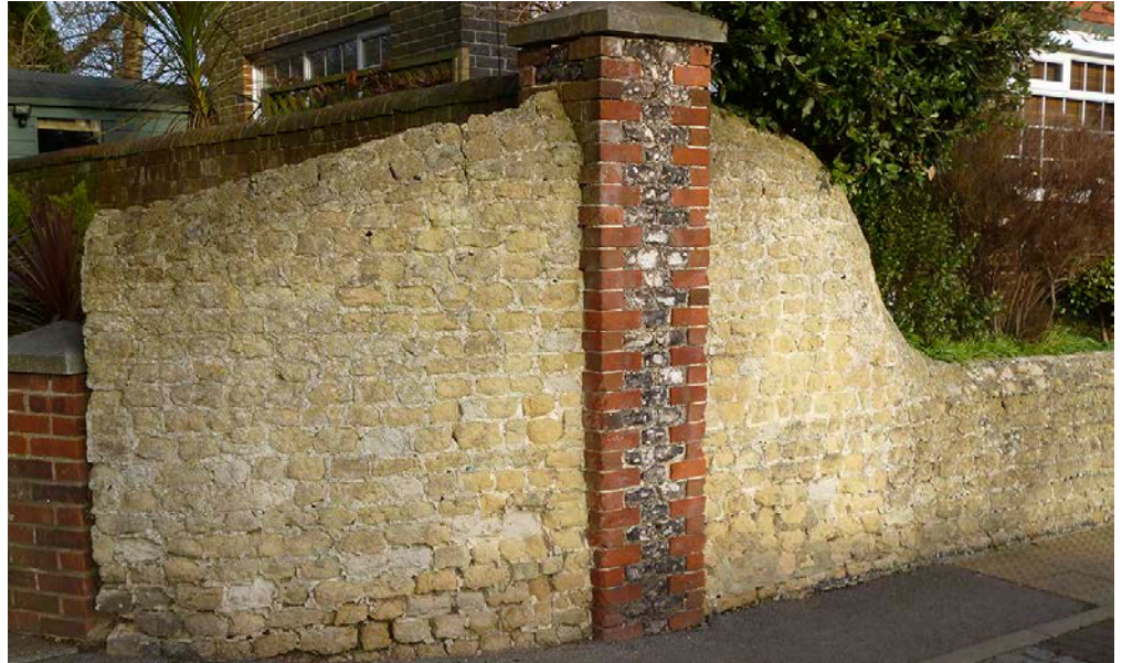
Figure 31: Garden wall, High Street, Langstone. Mixon Stone.
