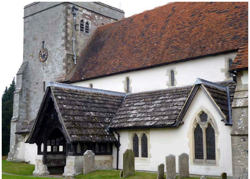
Figure 28: Porch and aisle, Holy Cross Church, Binsted. Horsham Stone slate tiles.
