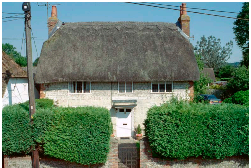
Figure 14: Cottage, Holybourne. Malmstone blocks (ground floor) and chalk block (first floor).
