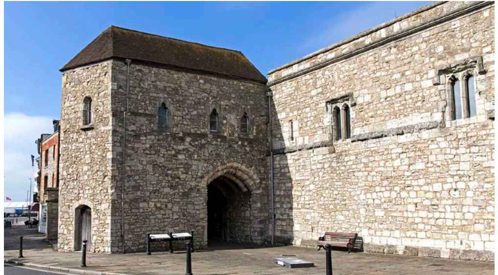
Figure 36: Gatehouse, Southampton. Bembridge Limestone with Sarsen stone, Bognor Rock, ferricrete and septaria.
