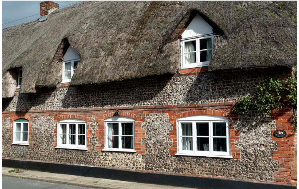
Figure 5: Hampshire downland thatched cottage. Flint nodules and rubblestone wall.
