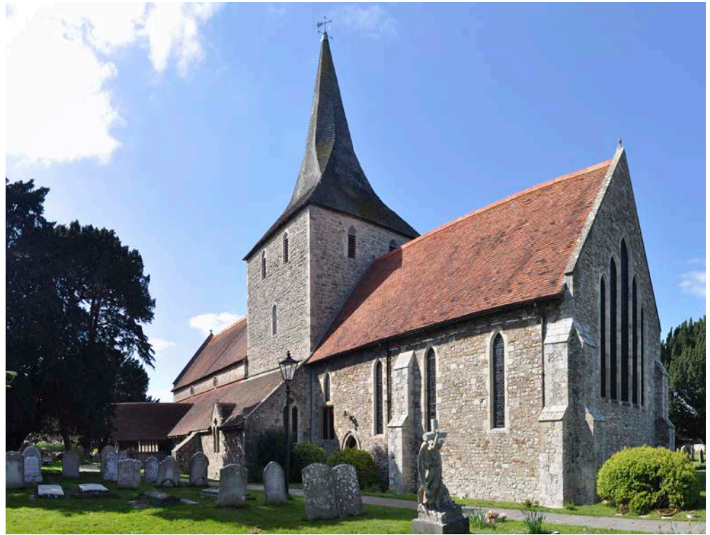
Figure 16: Church of St Mary, Hayling Island. Sarsen stone, Harwich Formation Siltstone, Beach Cobble Flint.
