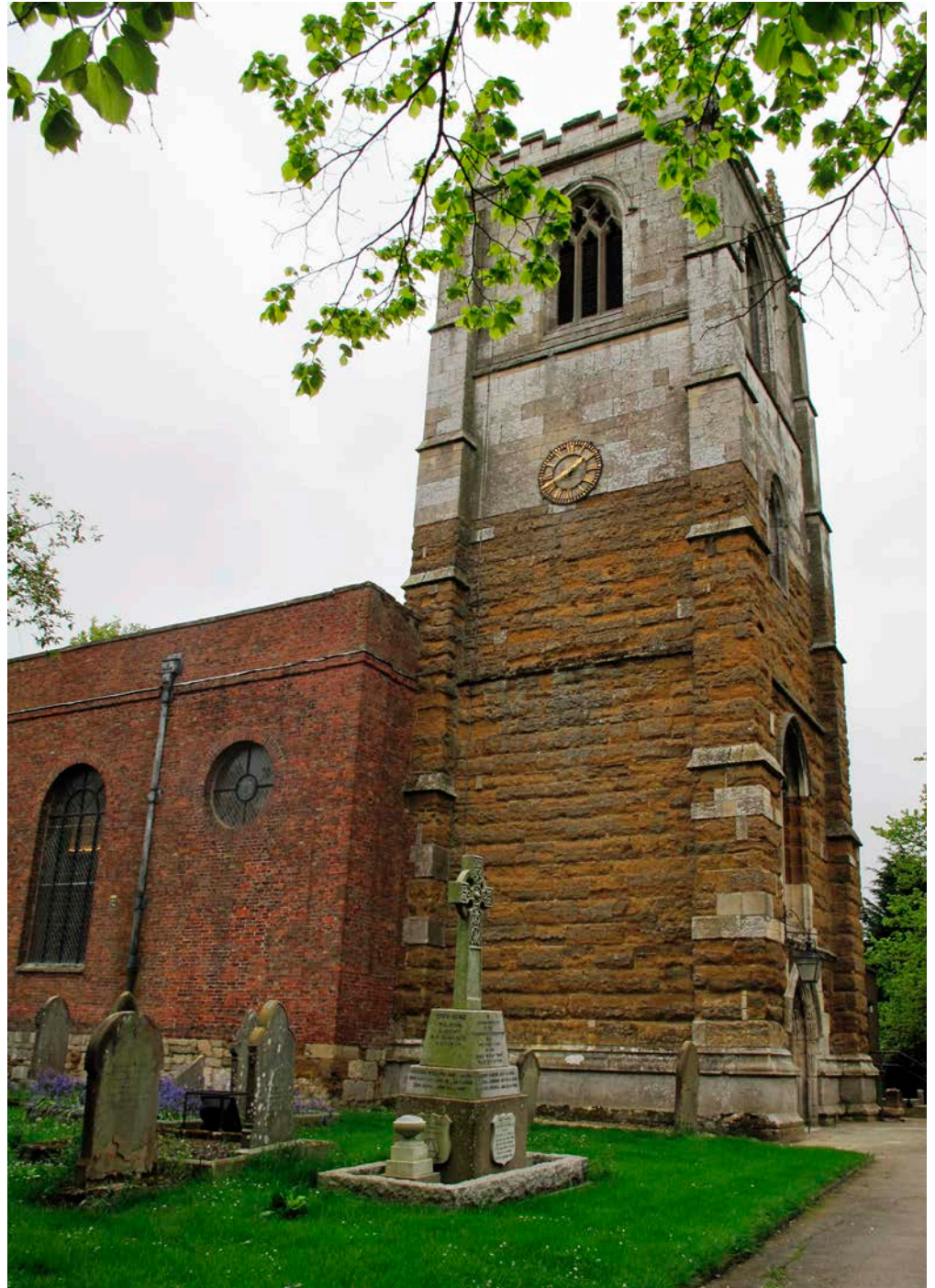
Figure 13: Church of St Peter, Humberston. Magnesian Limestone and reused Purbeck Marble.
