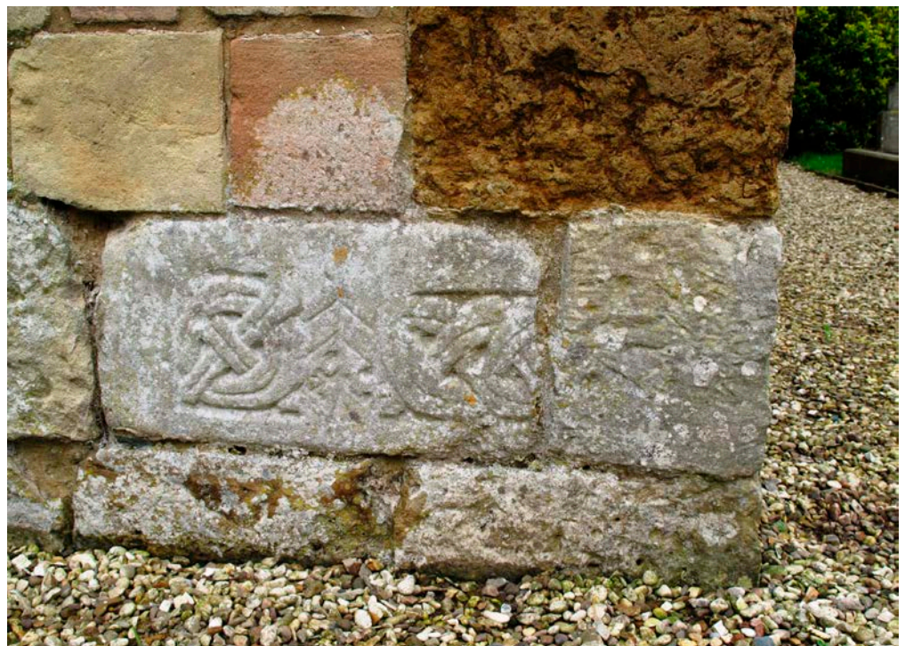
Figure 12: Tower footings, Church of St Peter, Humberston. Reused medieval Magnesian Limestone and Purbeck Marble.
