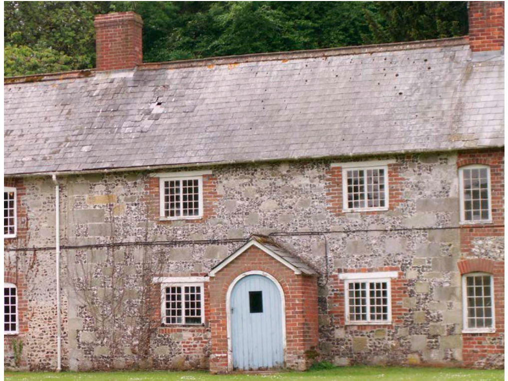
Figure 14: Terraced cottages, Tarrant Gunville. Flint, Upper Greensand chert and brick.
