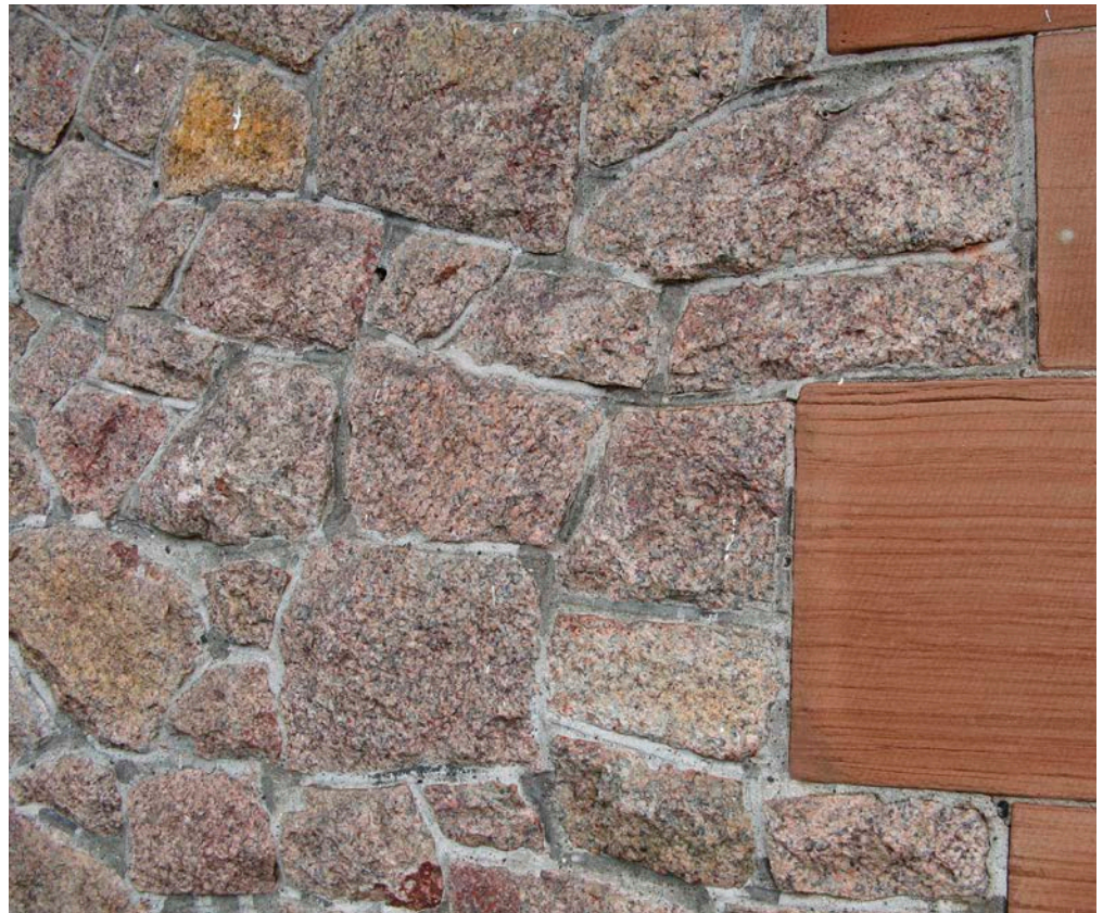
Figure 6: Railway station, Millom. Eskdale Granite blocks with dressings and bands of red-brown Sherwood Sandstone.
