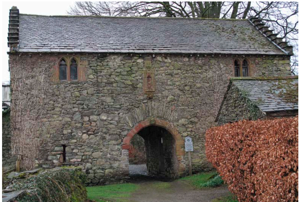
Figure 21: Hawkshead Old Courthouse, Ambleside. Borrowdale Volcanic Group rubblestone and boulders and Permo- Triassic sandstone.
