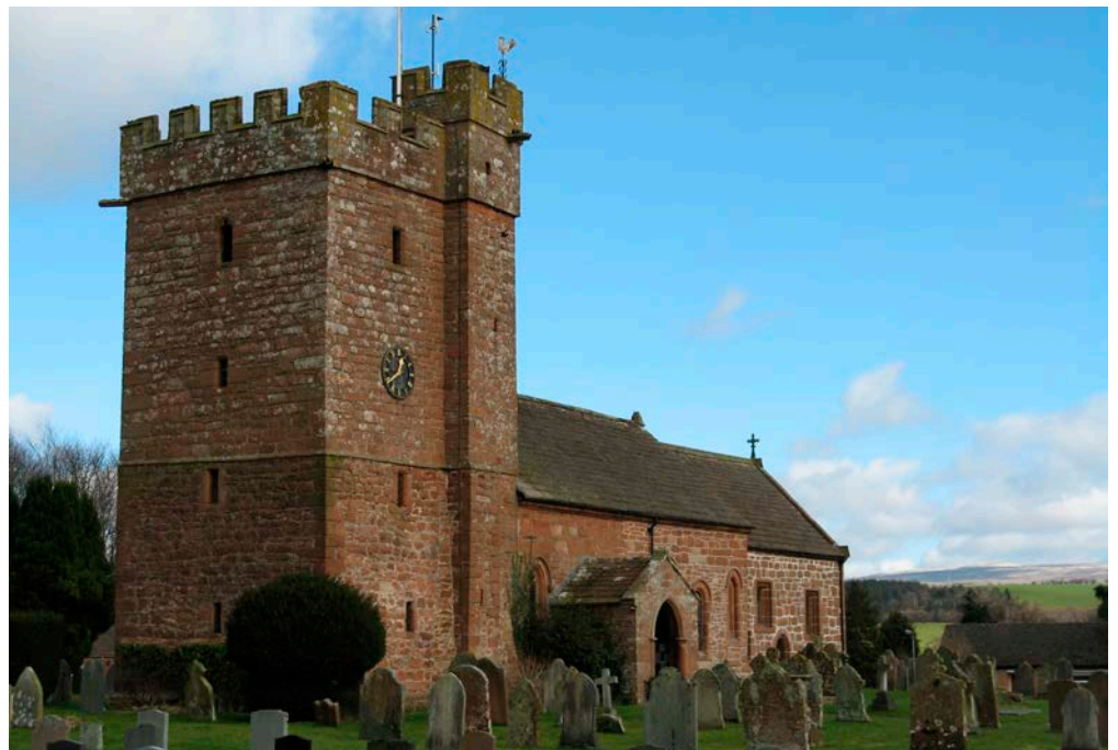
Figure 14: Church of St Cuthbert, Great Salkeld. Penrith Sandstone including roof.
