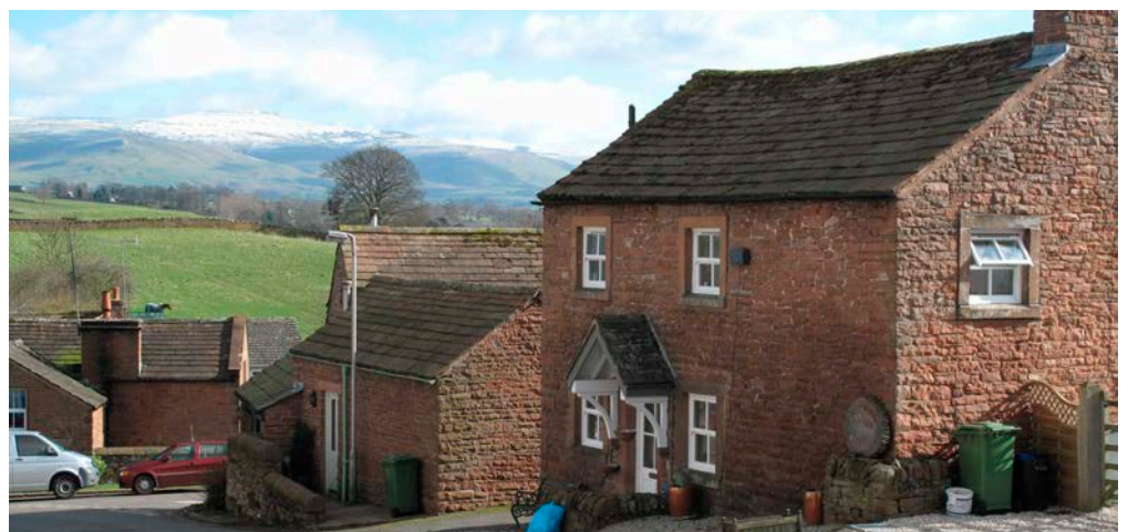
Figure 15: Houses and other buildings, Great Salkeld. Penrith Sandstone including roof slabs.
