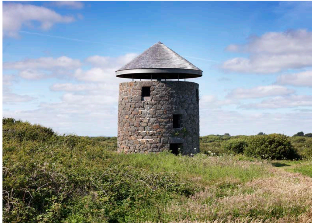
Figure 1: Tower mill ruin, Lizard Peninsula. Elvans and serpentinite.
