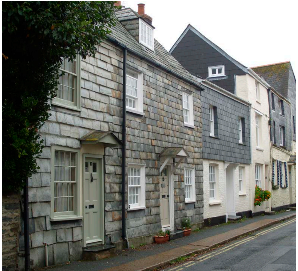
Figure 27: Church Street, Padstow. Delabole Slate and Carnglaze Slate fronts.
