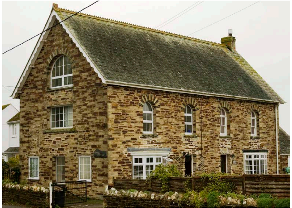
Figure 24: Former chapel, St Issey. St Issey Stone.
