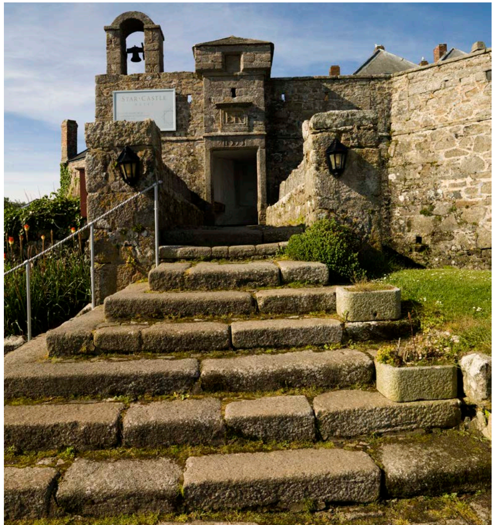
Figure 8: Star Castle, Hugh Town. Isles of Scilly Granite with slate roofs, including Delabole slate.
