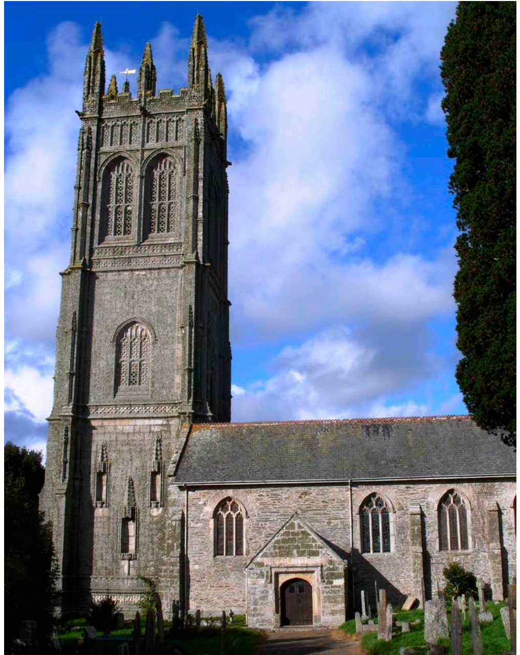
Figure 13: The Church of SS Probus and Grace, Probus. St Stephen's Stone Granite, and Delabole Slate roof.
