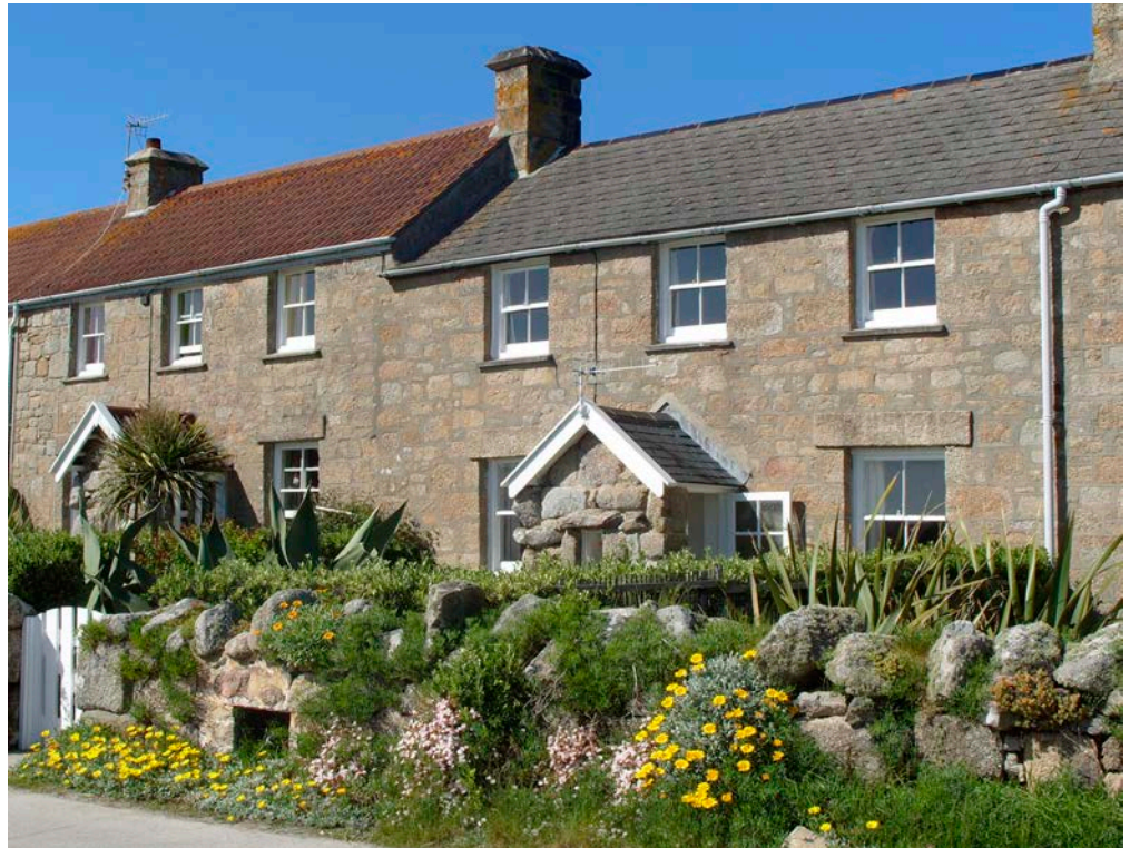
Figure 9: Cottages, Tresco. Tresco Granite.
