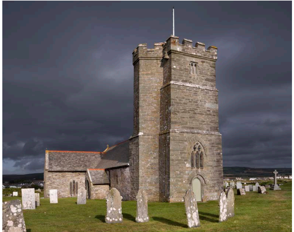
Figure 3: Church of St Materiana, Tintagel. Stone rubble including Greenstone, slate, hornblende and felspar.
