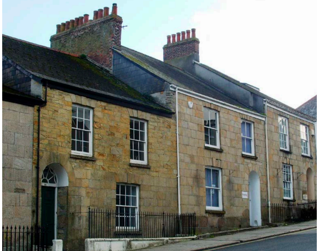
Figure 18: Houses, Lemon Street, Truro. Newham Stone.
