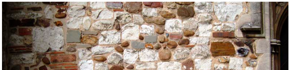
Figure 21: St George's Church, Toddington. Random rubble wall above Lower Greensand blocks.
