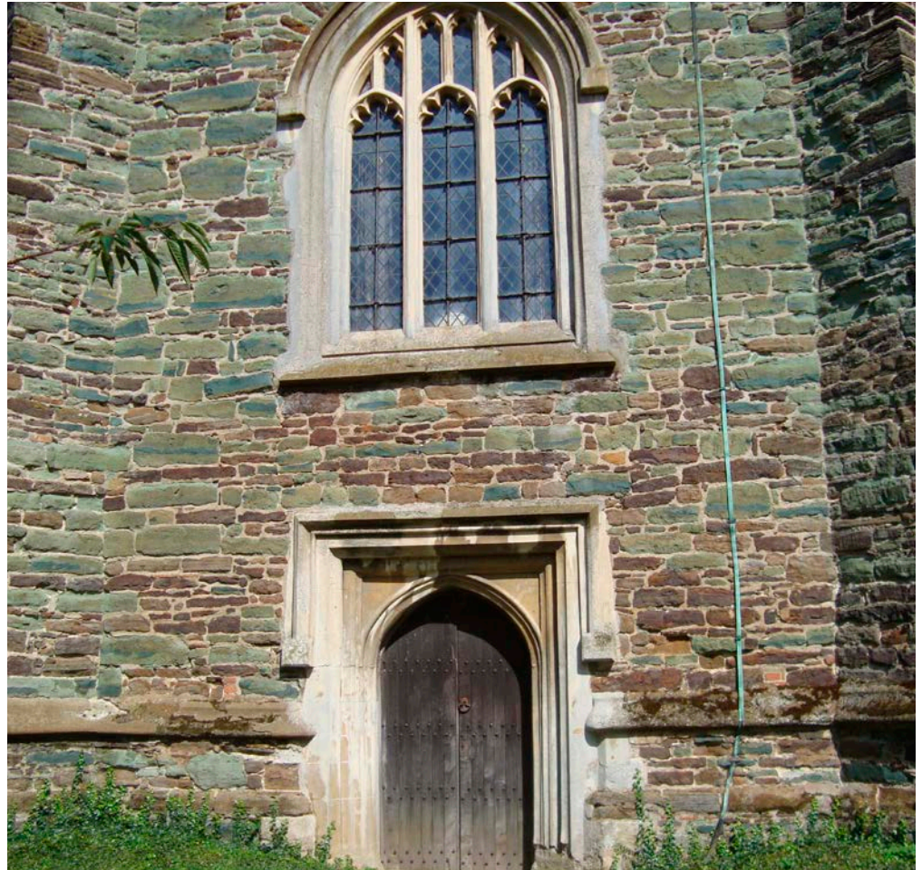
Figure 12: St James' Church, Husborne Crawley. Lower Greensand stone.
