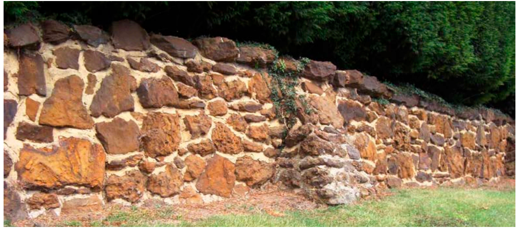
Figure 10: Wall near All Saints' Church, Tilsworth. Lower Greensand stone.
