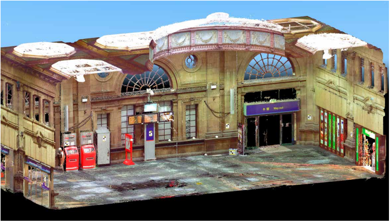
Figure CS2.1 Sectional view through the colourised laser scan point cloud of the listed ticket hall.
