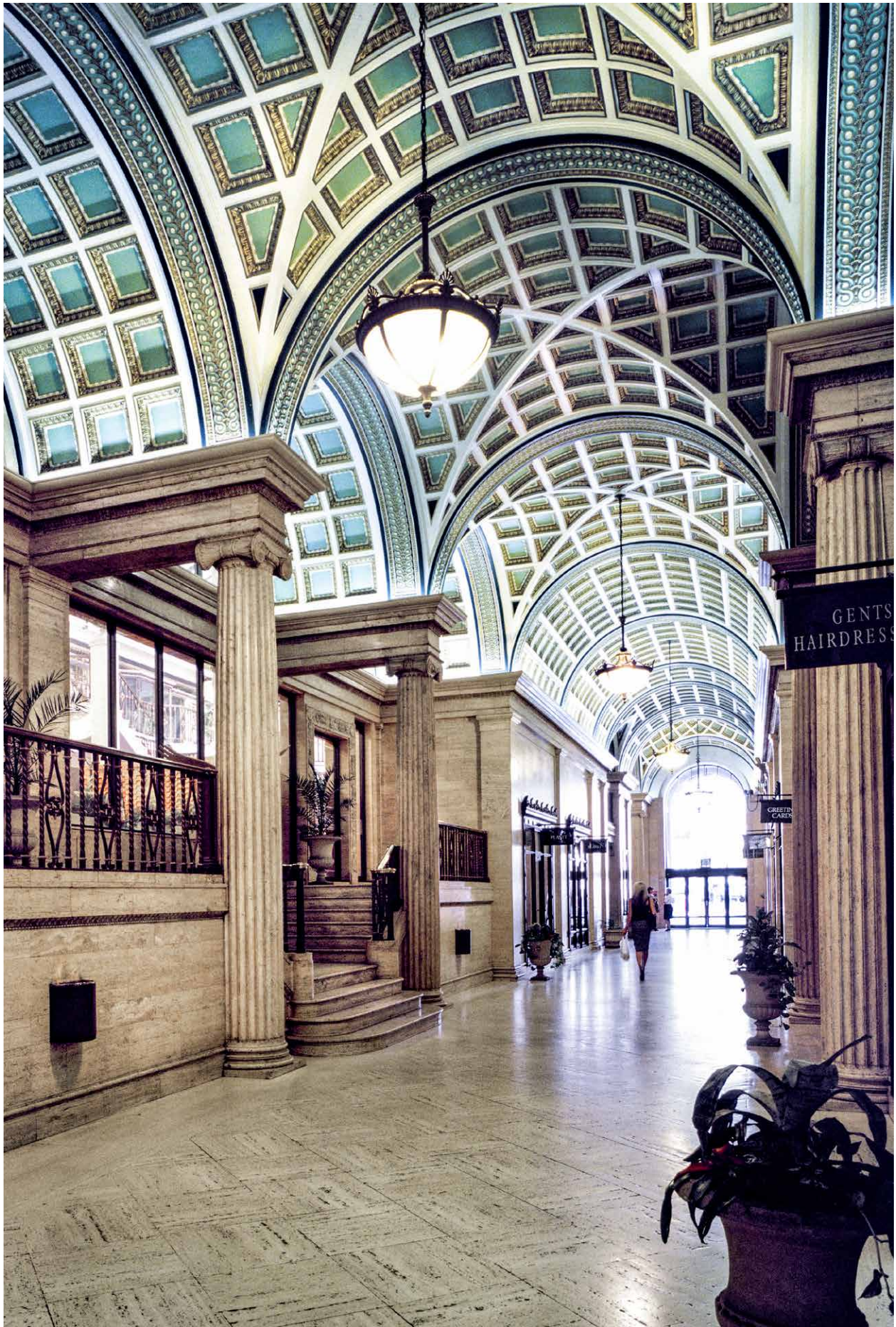
The internal arcade of India Buildings, Liverpool, being renovated as a Government Hub. © Historic England Archive
