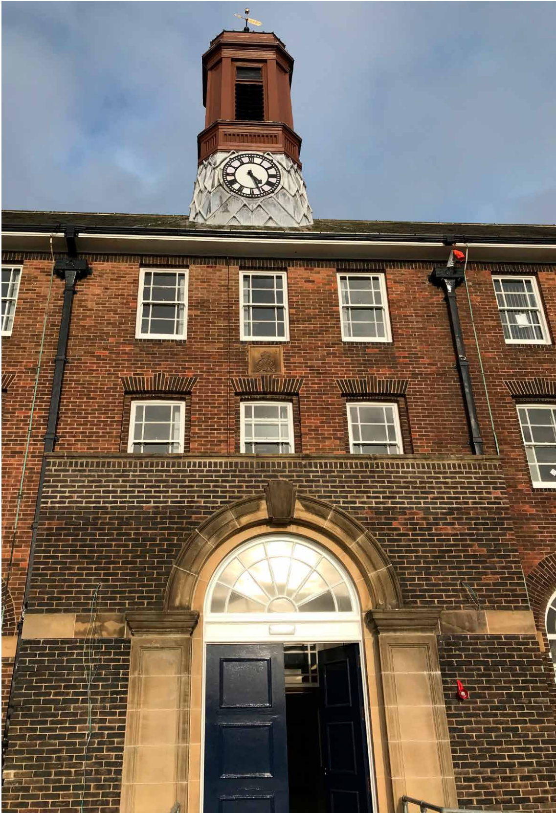
Sandhurst Block, Bourn Barracks, Catterick. This fine barrack block of 1938 has been renovated as offices with work to all the windows. © Crown Copyright
