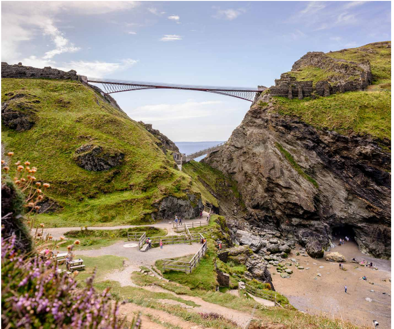
The new bridge at Tintagel Castle, Cornwall, is purposely designed to interfere as little as possible with the fabric and views. © Historic England / English Heritage Trust
