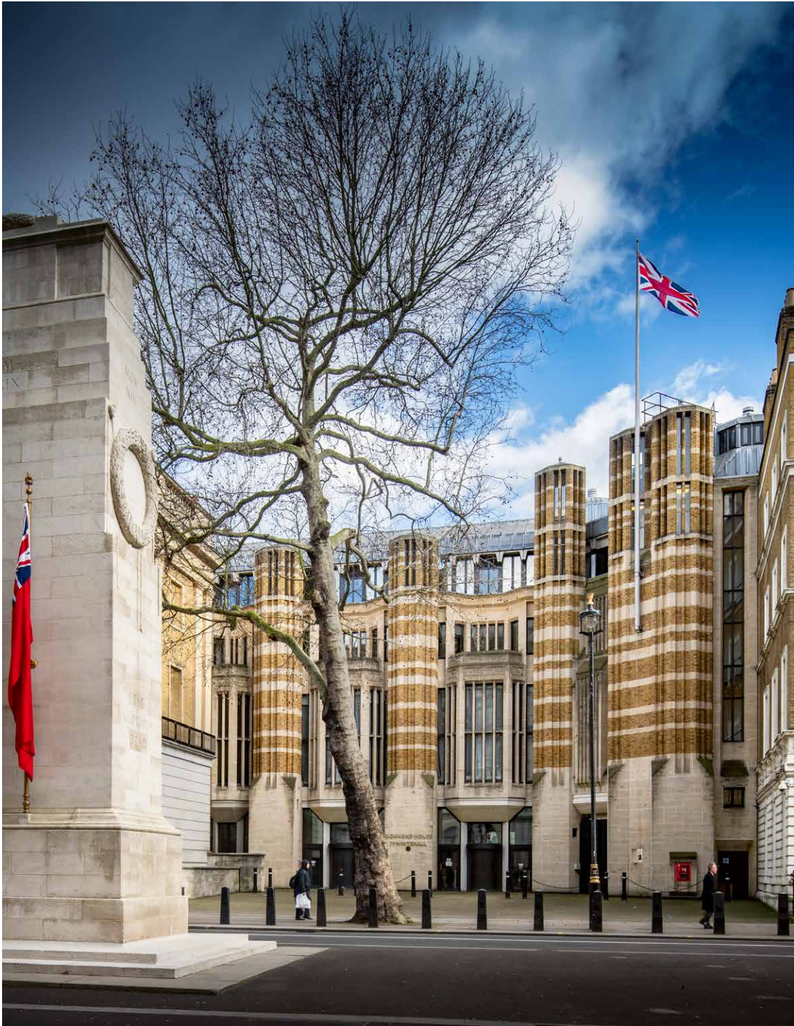
Richmond House, Greater London. Standing directly behind the Cenotaph, Richmond House (Grade II*) recently passed into the Parliamentary Estate. © Historic England Archive
