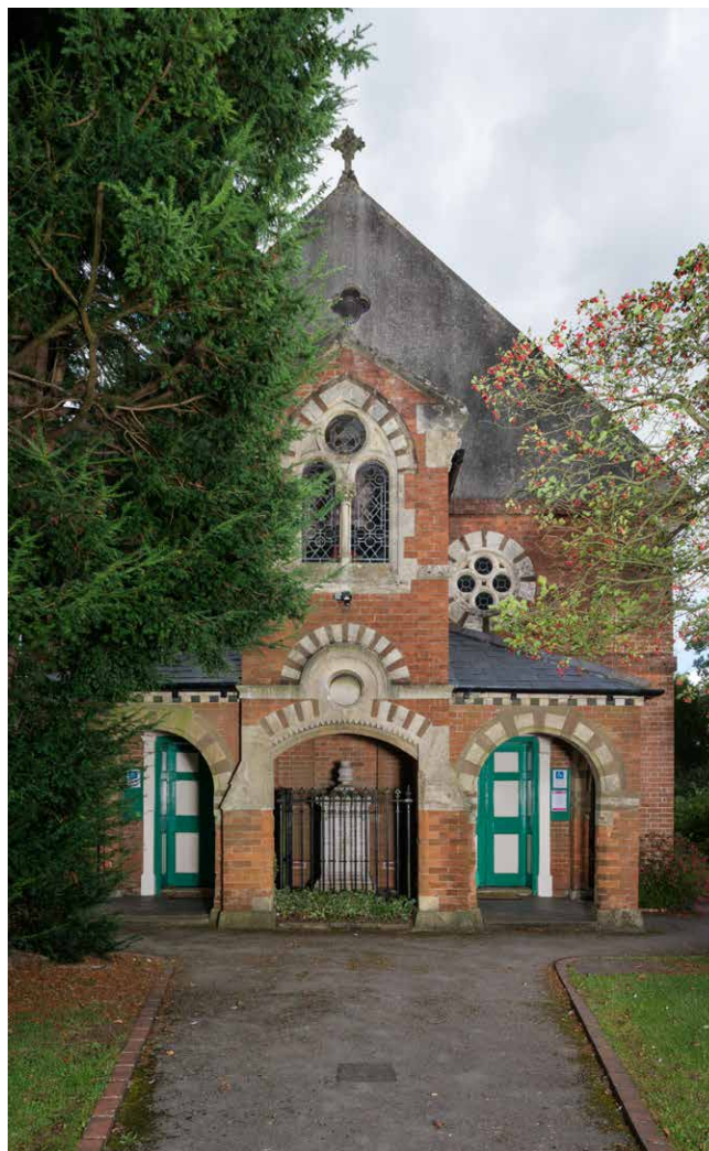
Kingswood Meeting House, Hollywood, Birmingham was awarded £26,400 by the Listed Places of Worship Roof Repair Fund to address urgent works to the roof. © Historic England
