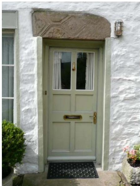
A very large carved stone re-used as a lintel to a smart doorway in Dent. ©YDNPA
