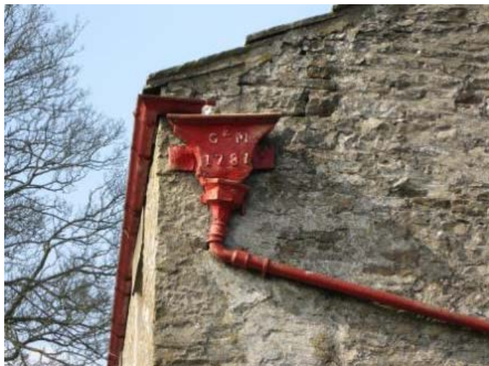
With lead vulnerable to theft today, finding the original 1781 lead hopper still in place is a significant heritage asset to the Dales. © YDNPA
