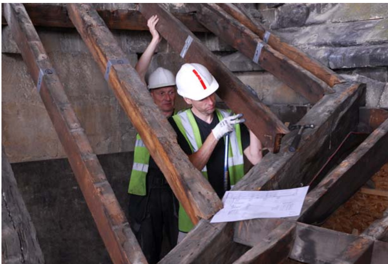
Figure 2- Jason Varnam, HLF Skills for the Future Bursary student (right) working with Carpentry mentor Stuart Cook easing a rafter from the valley beam on Lincoln Cathedral © Lincoln Cathedral Works Department.
