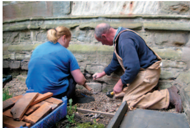
Anthony Goode demonstrating tile repairs at Holy Trinity Church, Radcliffe. © SPAB
