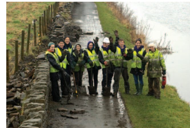
Dry stone walling, Leeds/Liverpool canal in Rhiston, March 2011. © Waterways Action Squad
