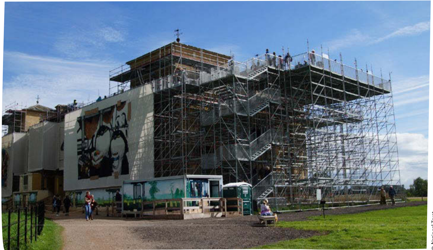
Above View of scaffolding and entrance hub
