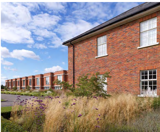
Former officers mess building (foreground) and new terrace beyond
