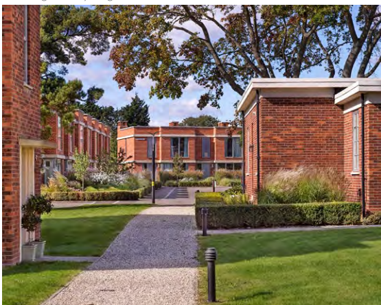
Retained military buildings (foreground) and new terraces beyond
